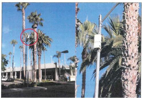
Figure 2: Small cell (in red circle) mounted on an existing light standard [Close up on right].
