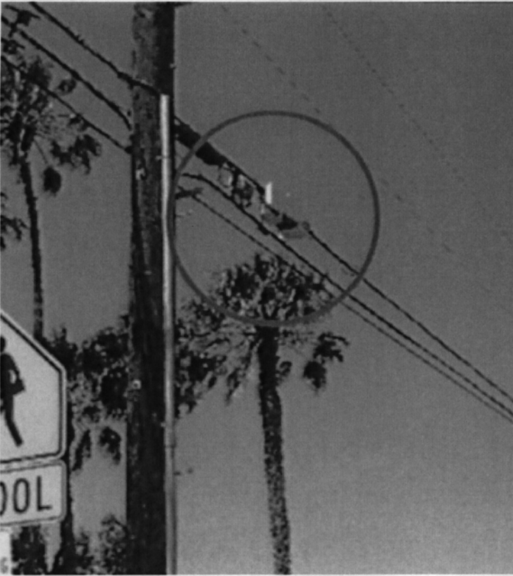
Small cell (circled in red) on a pole-to-pole strand in Torrance, California; at right, a small cell mounted onto a pre-existing light standard. Photographs courtesy of the City of Pasadena
