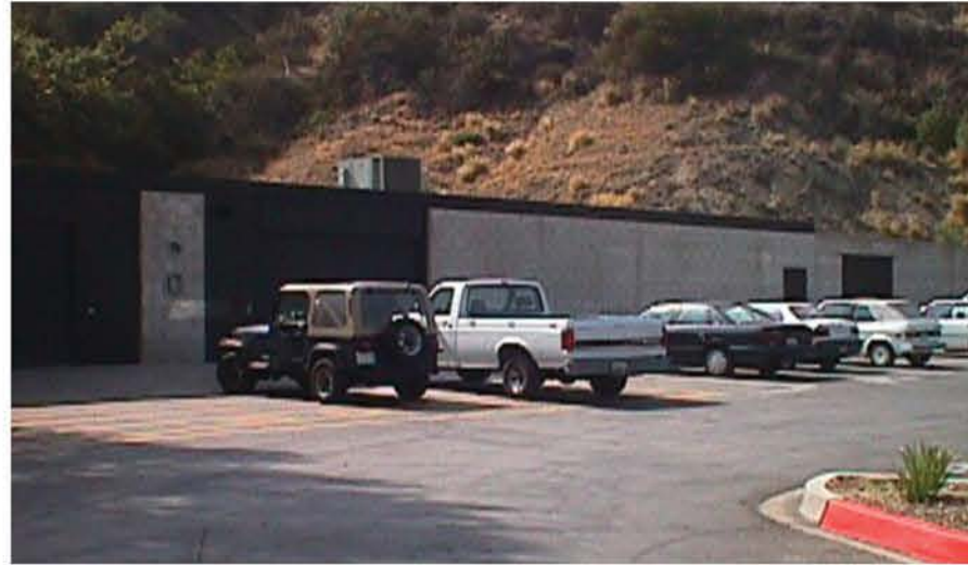
EXTERIOR VIEW / SOUTH BUILDING
