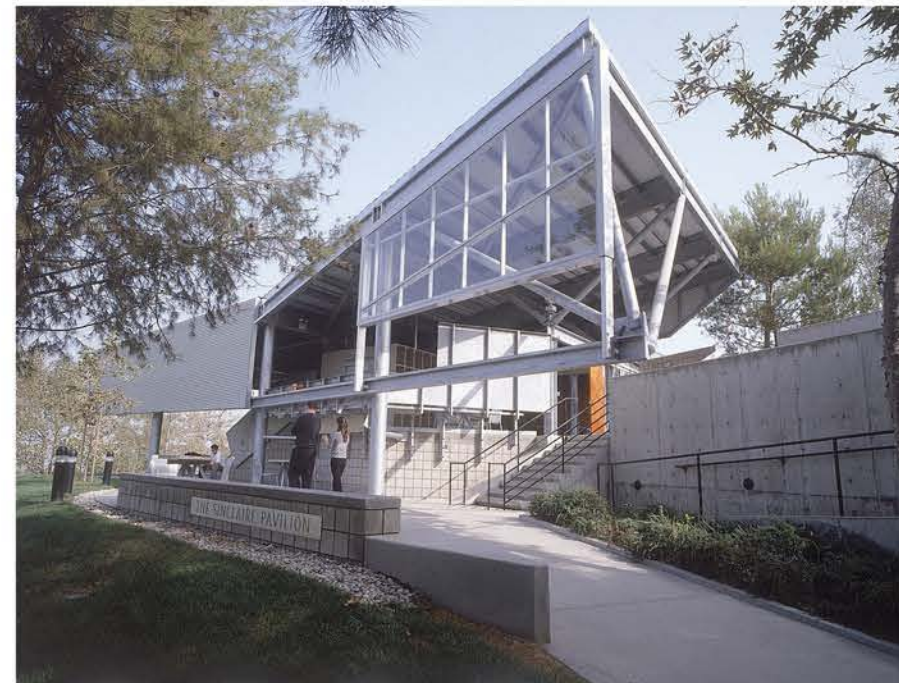
EXTERIOR VIEW / SINCLAIRE PAVILION
