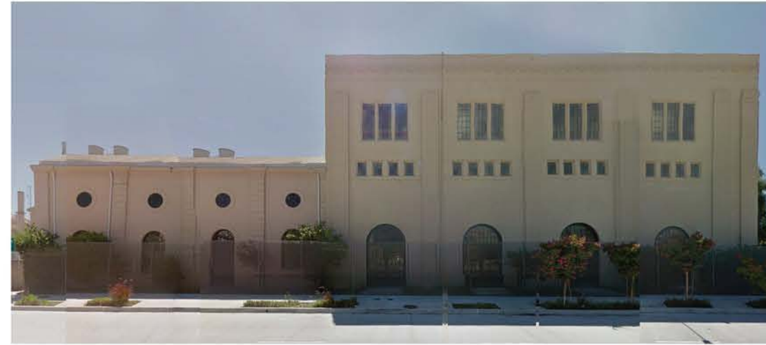
C / GLENARM POWER PLANT
