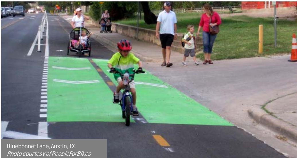
FIGURE 4-3 GREEN PAINT PERPENDICULAR TO DRIVEWAY
