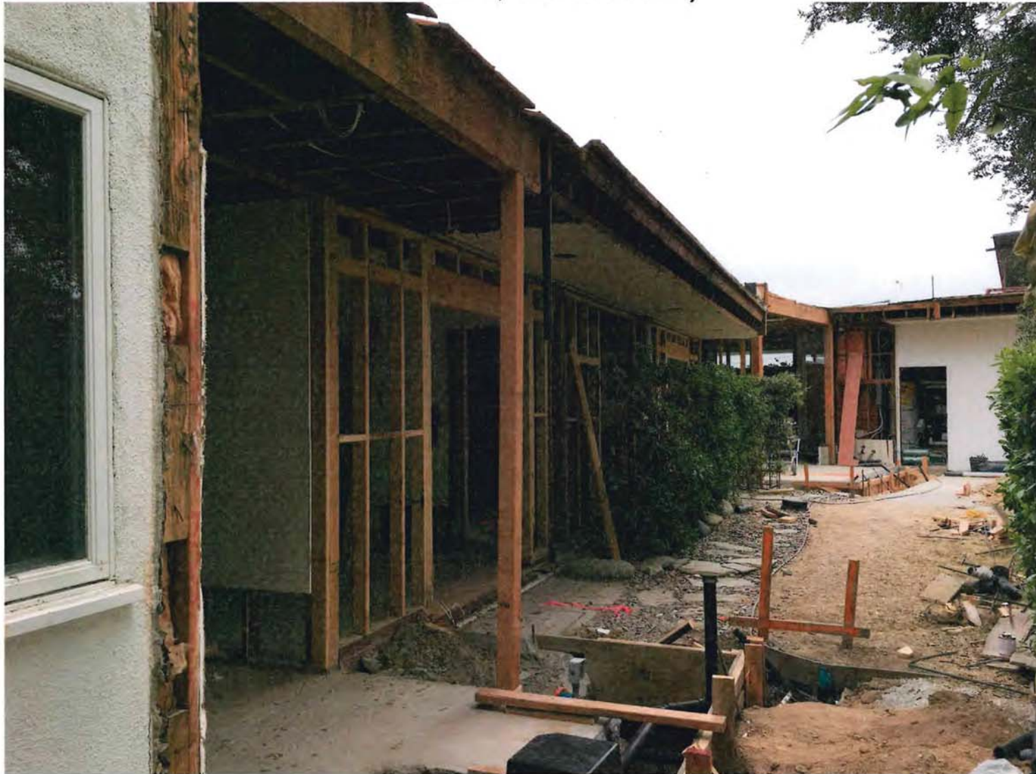
Attachment C: 95 Tustin Road: Portion of West Elevation (1994 Additions; June 2017)
