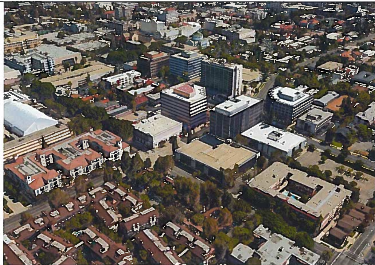
EXISTING CONDITION - SW AERIAL
