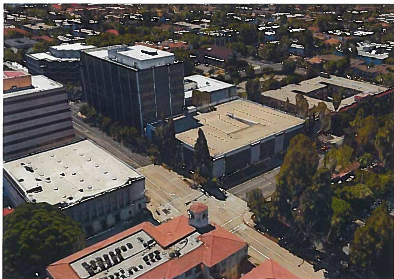
EXISTING CONDITION - NW AERIAL
