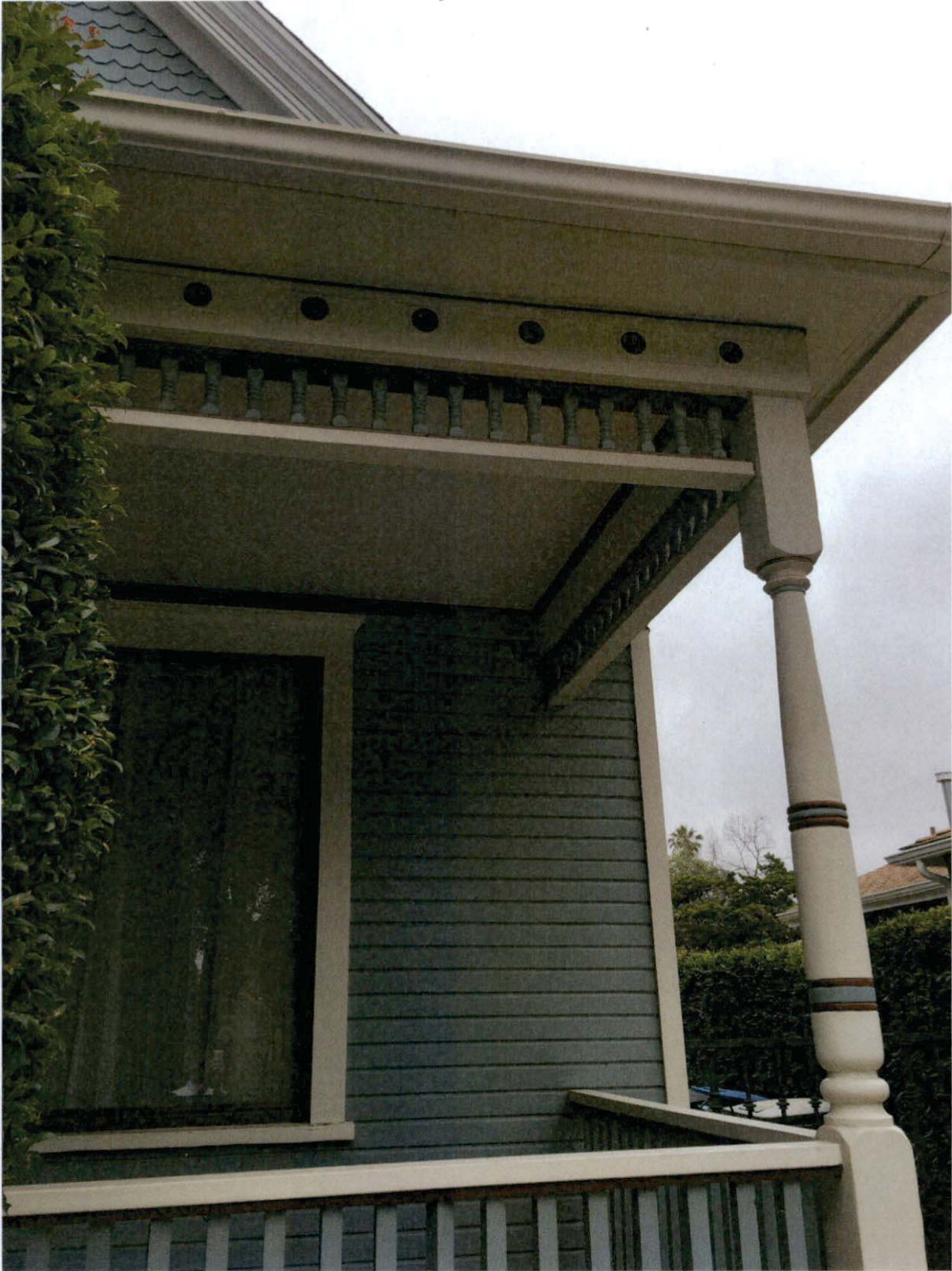
Current Photographs: South Elevation; Porch Post/Frieze/Spindlework Detail
