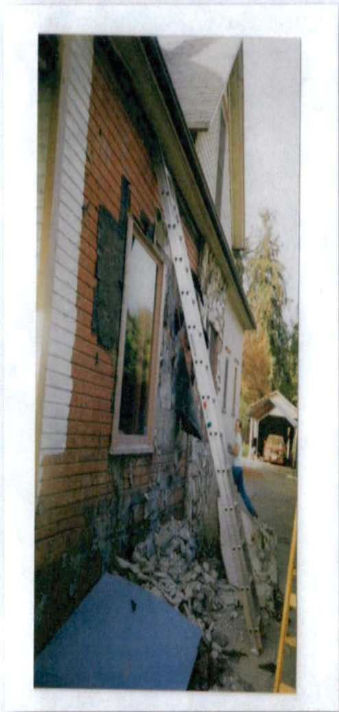
In addition to the work on the front of the home, they removed stucco from the side of the house, which revealed the home's original wood siding.
