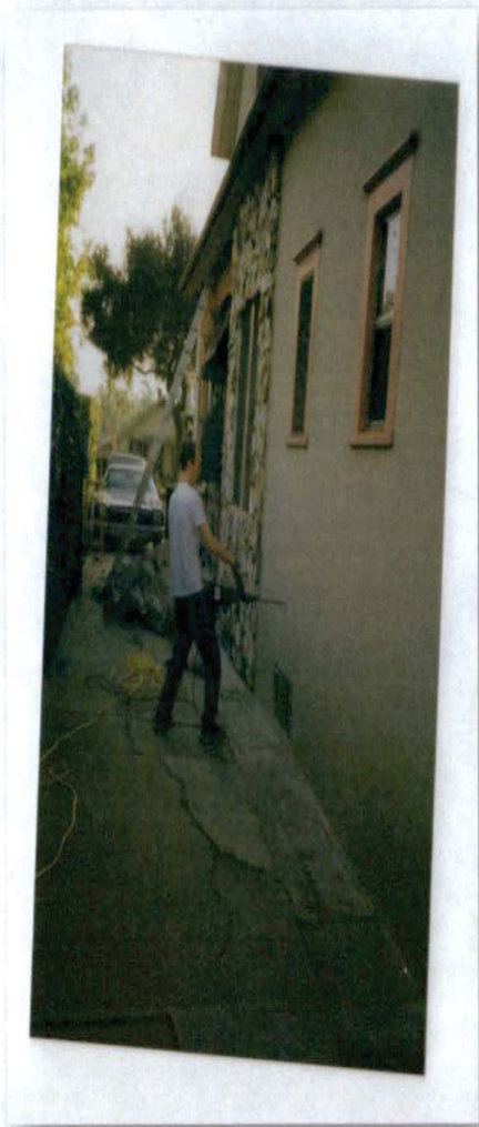
In addition to the work on the front of the home, they removed stucco from the side of the house, which revealed the home's original wood siding.
