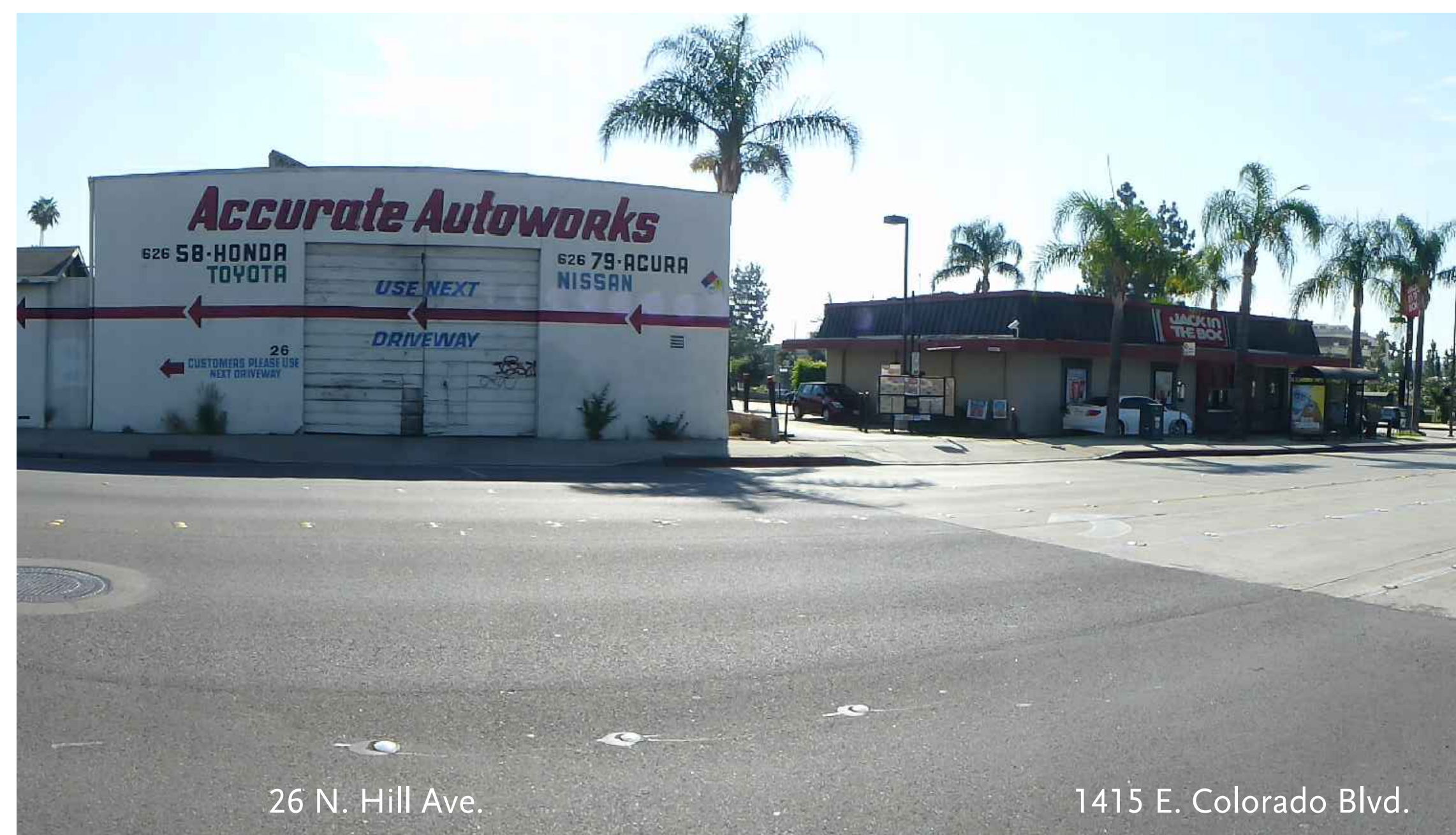
View of the buildings on the opposite side of Hill Ave. from the North Parcel site. 6
