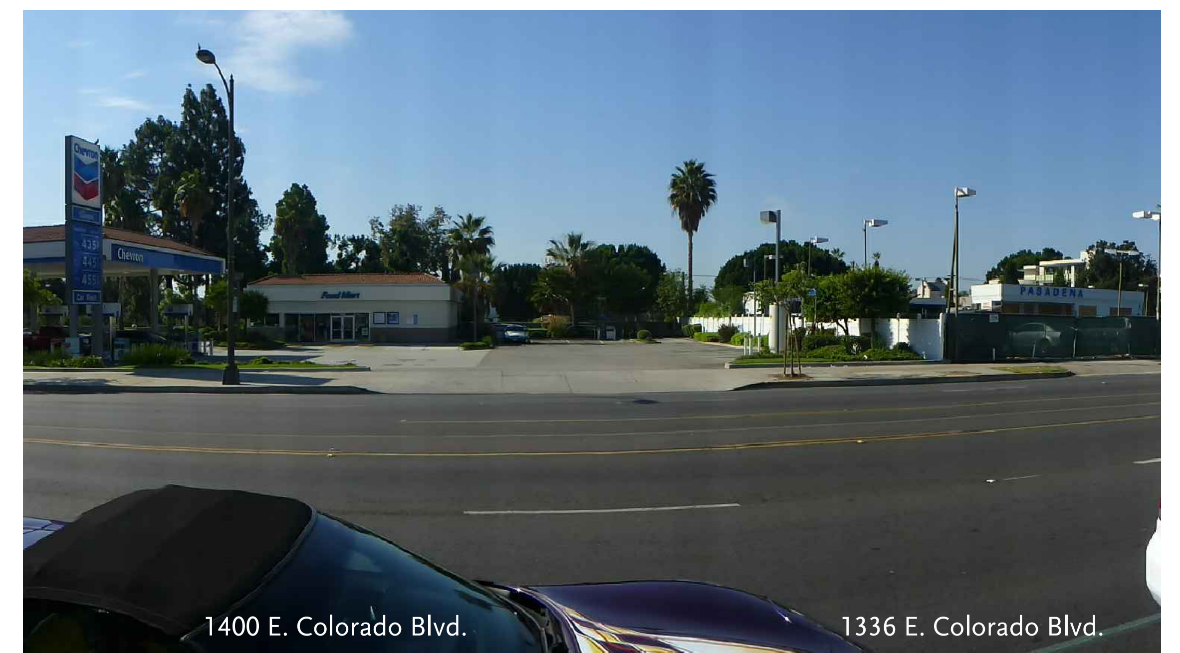
View of the South Parcel site and neighboring gas station from Colorado Blvd. 3
