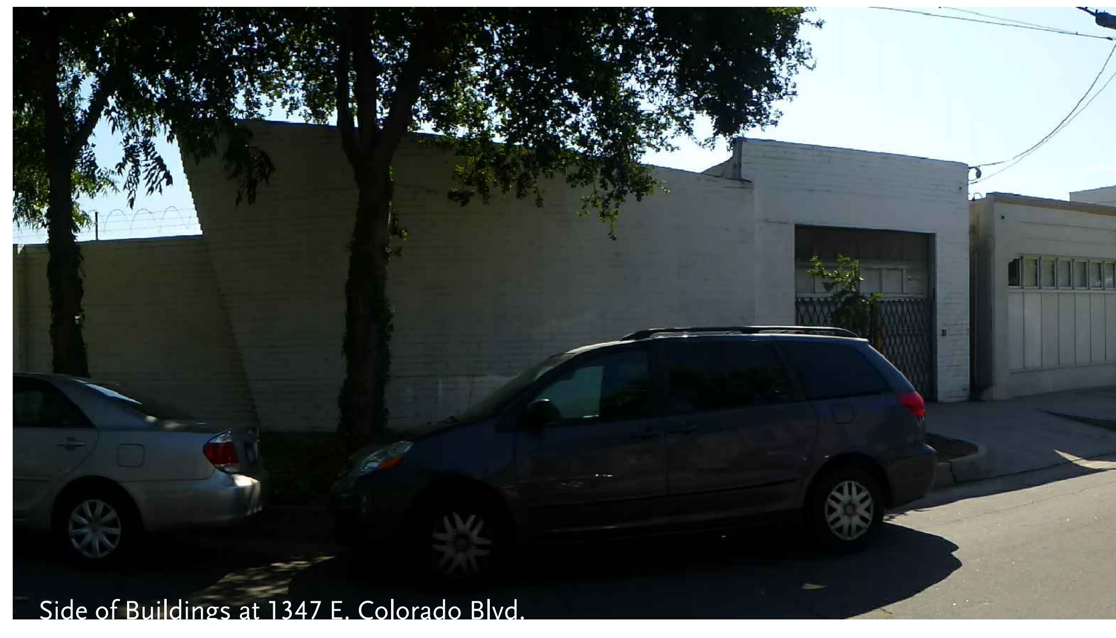
View of existing buildings on North Parcel site from Holliston Ave. 5
