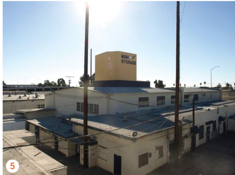
5 BUILDINGS 05 : STORAGE FACILITIES AND SILO
