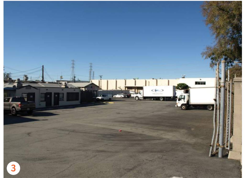
3 BUILDINGS 09(LEFT) & 30(BEYOND) : STORAGE FACILITIES AND OFFICES
