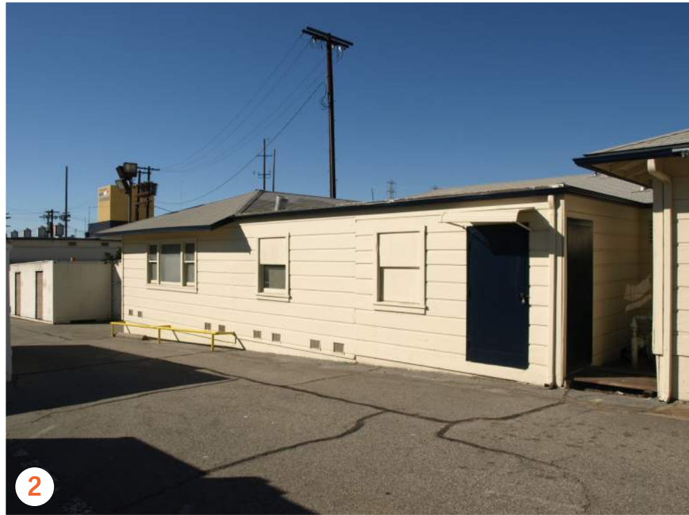
2 BUILDING 10 : STORAGE FACILITIES
