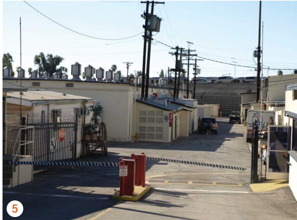
BUILDINGS 10(LEFT) & 03(MIDDLE) : STORAGE FACILITIES
