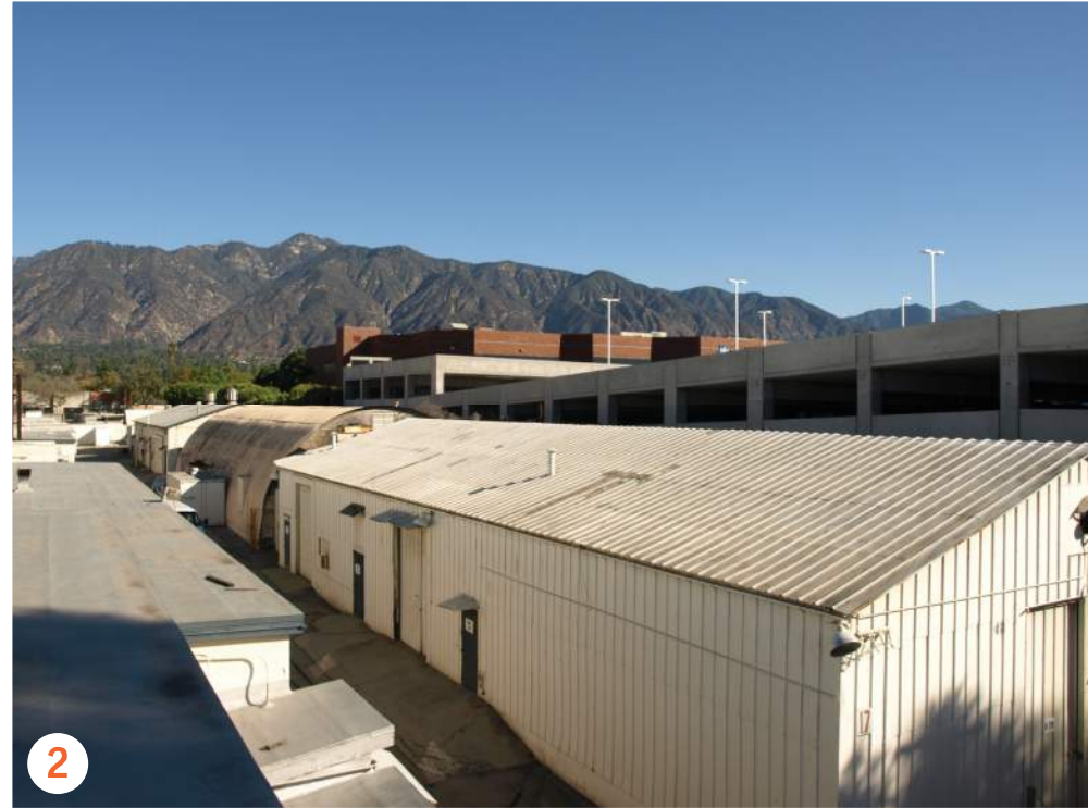
BUILDING 14 : STORAGE FACILITIES
