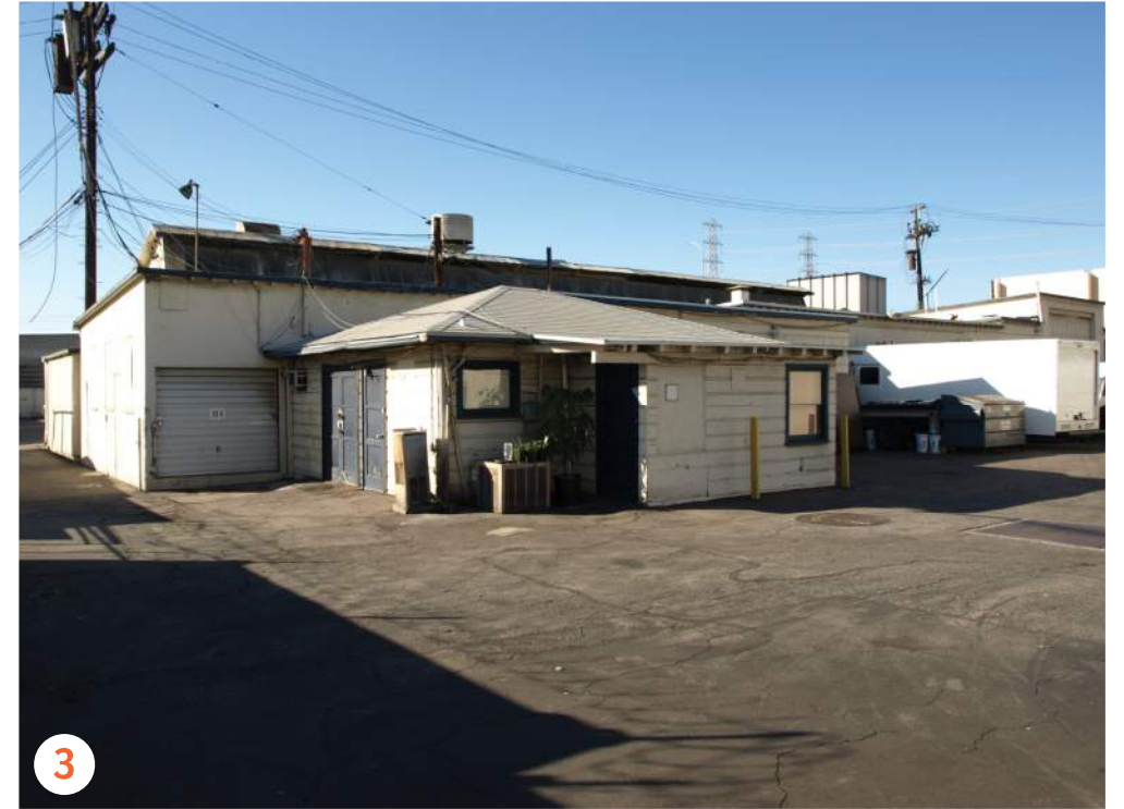
3 BUILDING 11 : STORAGE FACILITIES
