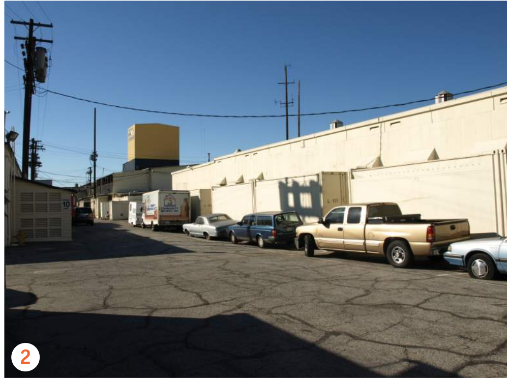
BUILDING 14 : STORAGE FACILITIES
