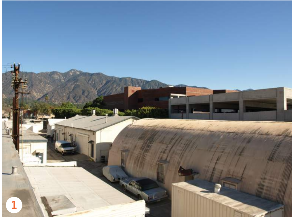
BUILDING 12(RIGHT) & 02(MIDDLE) : STORAGE FACILITIES
