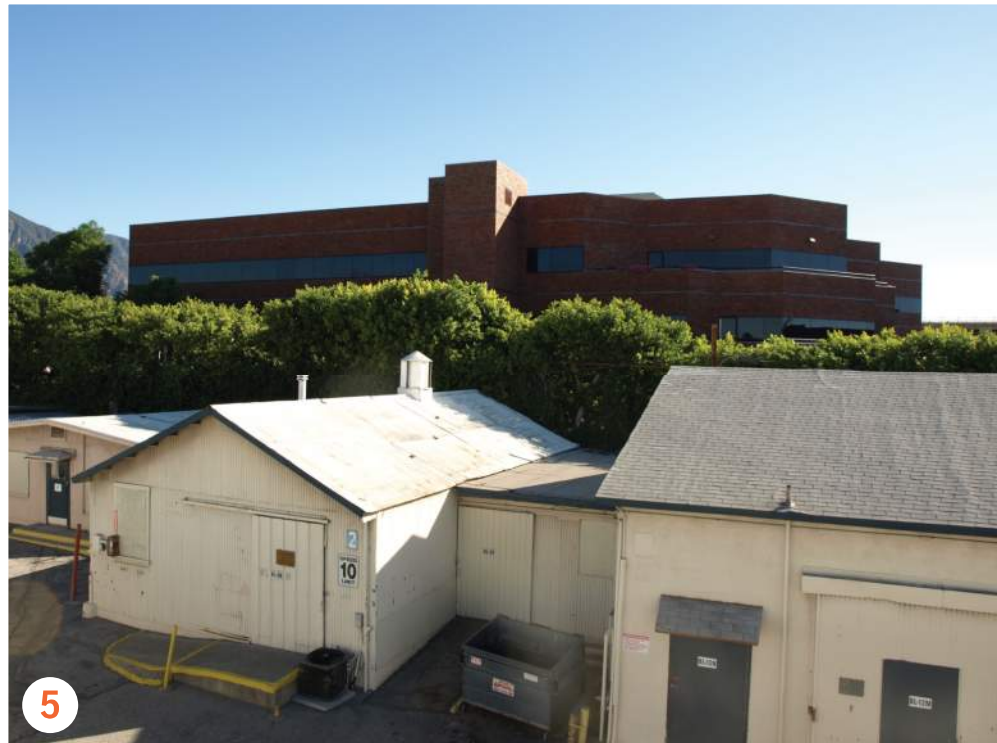
5 BUILDINGS 01(LEFT) & 02(RIGHT) : STORAGE FACILITIES
