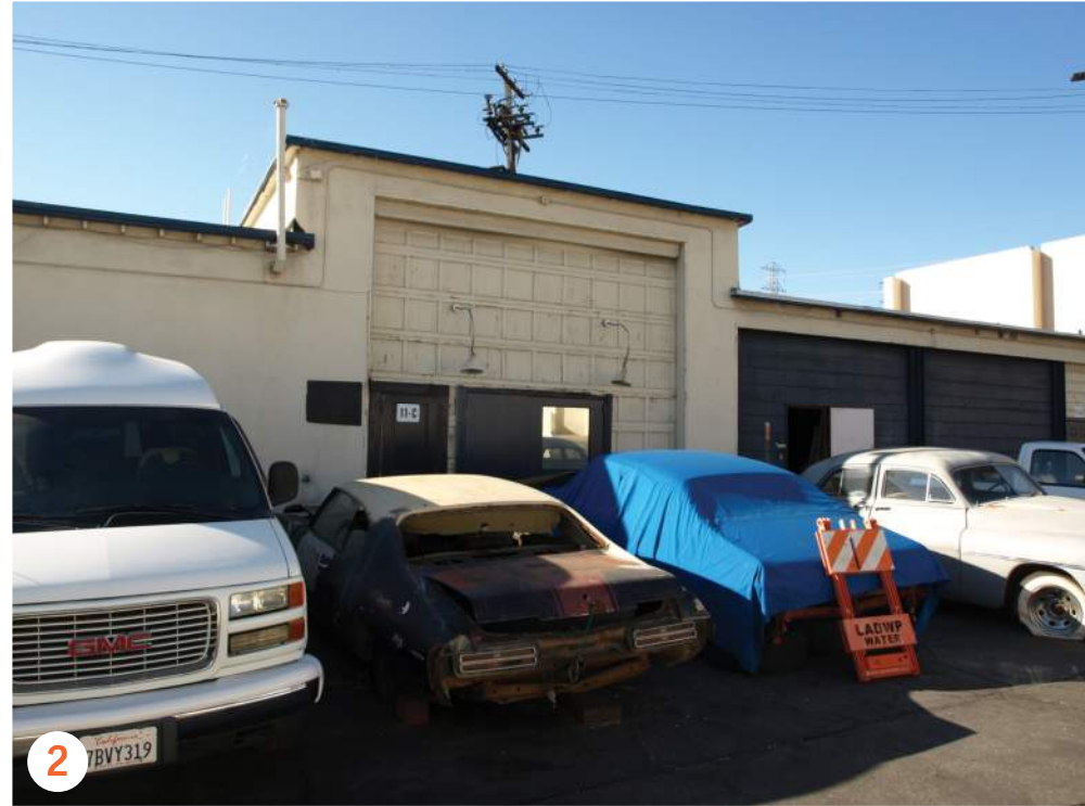
2 BUILDING 11 : STORAGE FACILITIES
