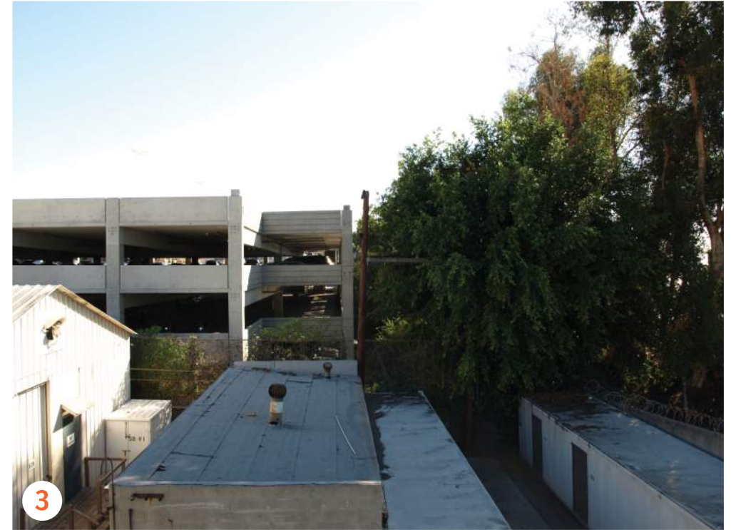
BUILDING 17 : STORAGE FACILITIES
