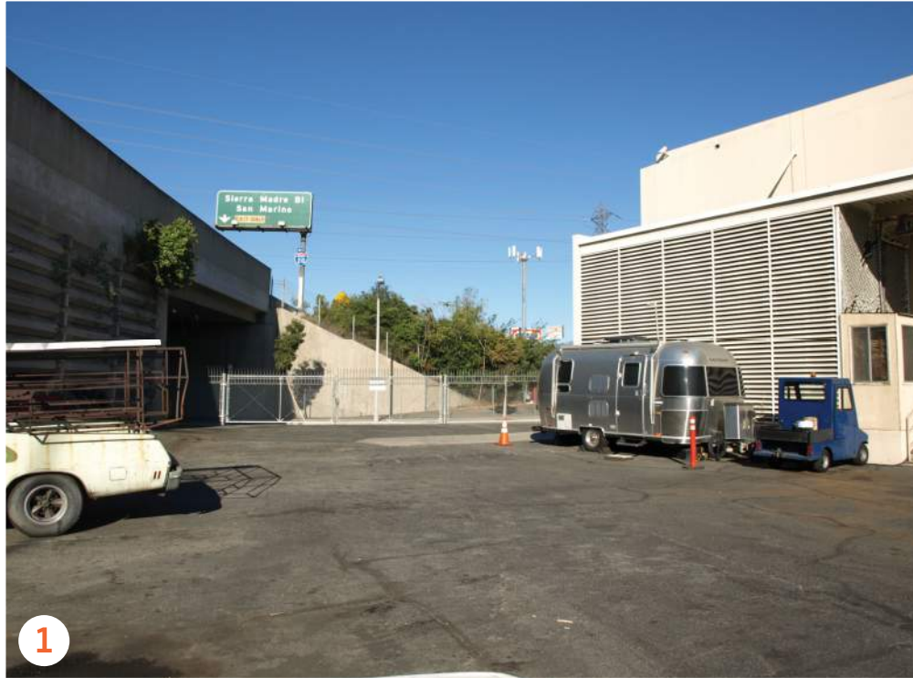
1 BUILDING 30 : OFFICE BUILDING AND WAREHOUSE(RIGHT)
