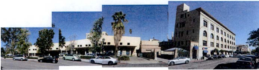
4. VIEW EAST FROM OAKLAND, SOUTH OF UNION
