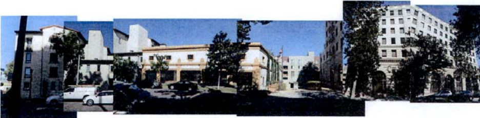
2. VIEW EAST FROM MADISON, SOUTH OF UNION
