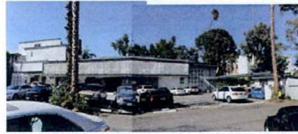
15. VIEW NORTH FROM PARKING LOT ON NW CORNER OF UNION AND MADISON
