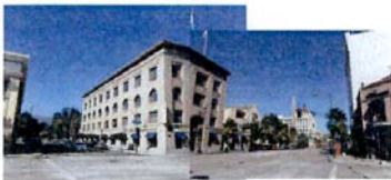
3. VIEW NORTH FROM COLORADO
