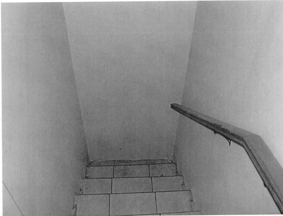
Figure 15. Looking south down the second-story stairs ending in a sealed wall closed off to the first floor.
