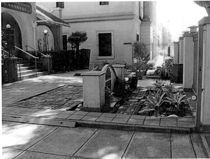
Figure 12. Looking south at the front yard area with modern Mexican tile porch pavers, concrete paving, red brick, and square piers with sign.
