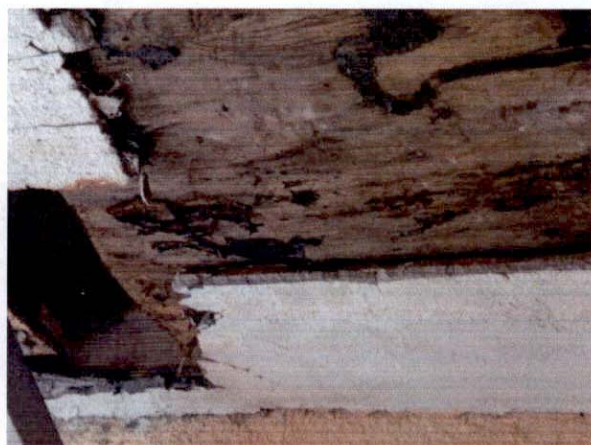
Figures 5 & 6: Termite Damage to Porch Entry Soffit
