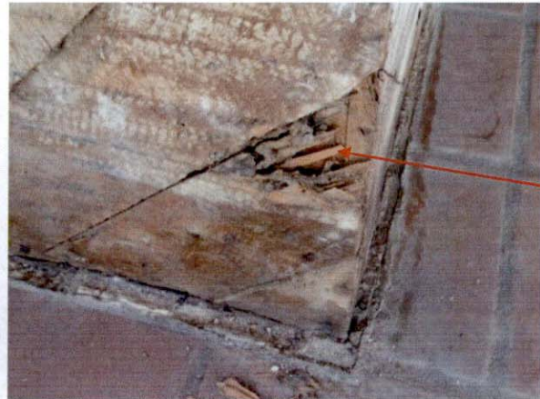
Figures 1 & 2: Termite Damage to Wall Sheathing at Porch Entry (Looking East)
