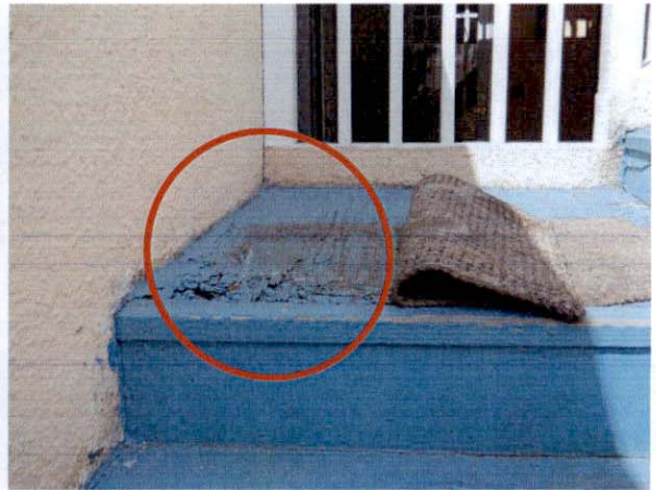
Figures 18 & 19: Damage at Rear Stair Landing & Walkway (Looking South & West)
