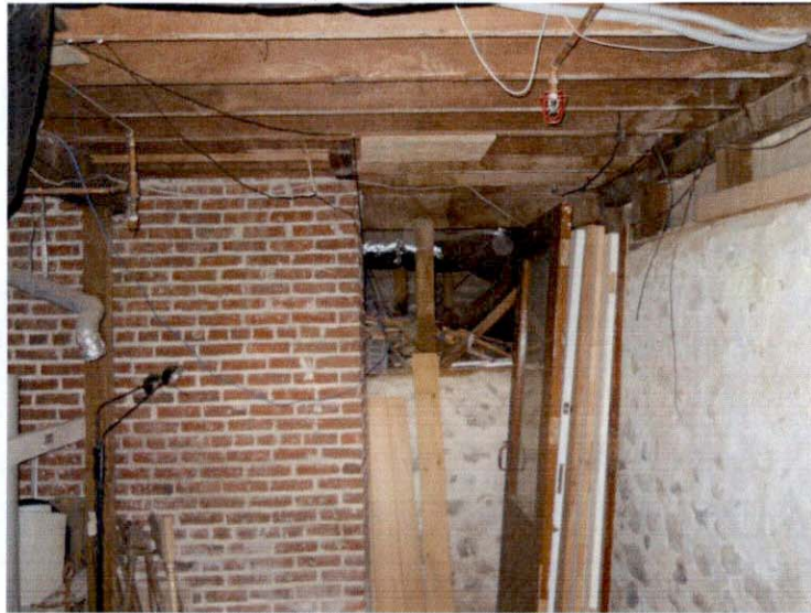
Figure 14: Brick Chimney at Foundation (Looking South)
