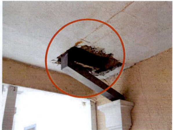
Figures 17 & 18: Damage at Rear Stair & Soffit (Looking East)
