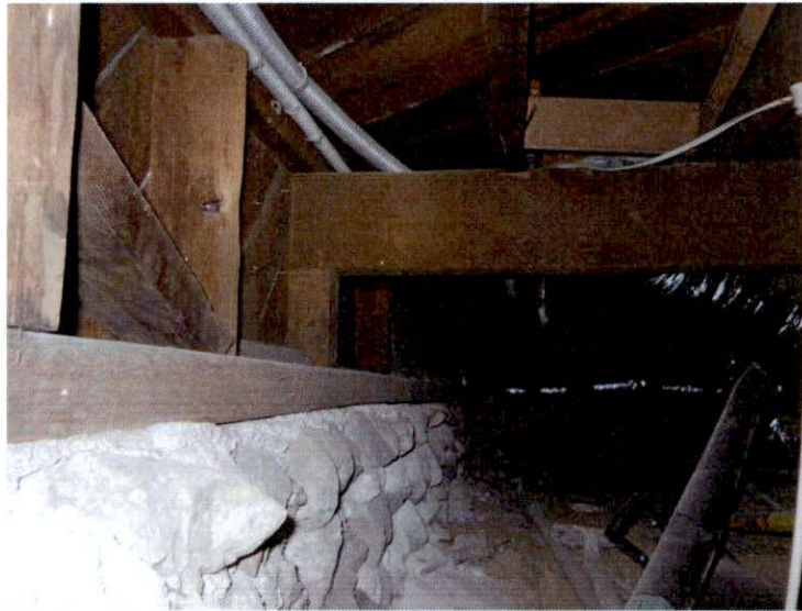
Figure 11: Typical Foundation Without Anchorage (Looking South)
