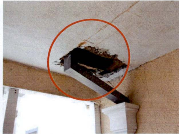
Figures 16 & 17: Damage at Rear Stair & Soffit (Looking East)
