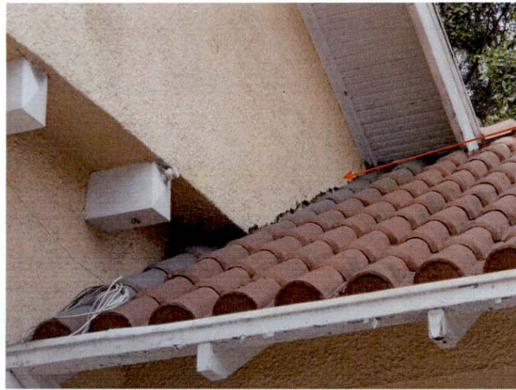
Figure 5: Spalling at Entry Roof (Looking Southwest)
