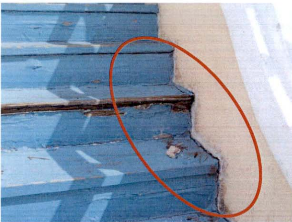
Figures 20 & 21: Damage at Rear Stair & Walkway (Looking North & South)
