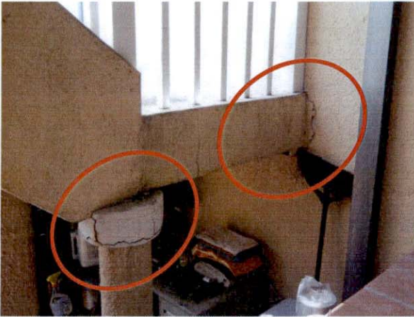
Figures 16 & 17: Damage at Rear Stair & Soffit (Looking East)
