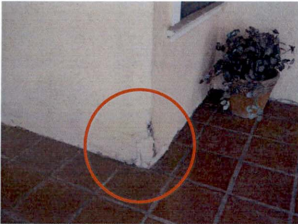
Figures 1 & 2: Termite Damage to Wall Sheathing at Porch Entry (Looking East)
