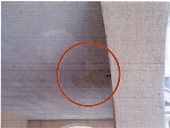
Figures 3 & 4: Termite Damage to Wood Lath at Porch Entry Soffit
