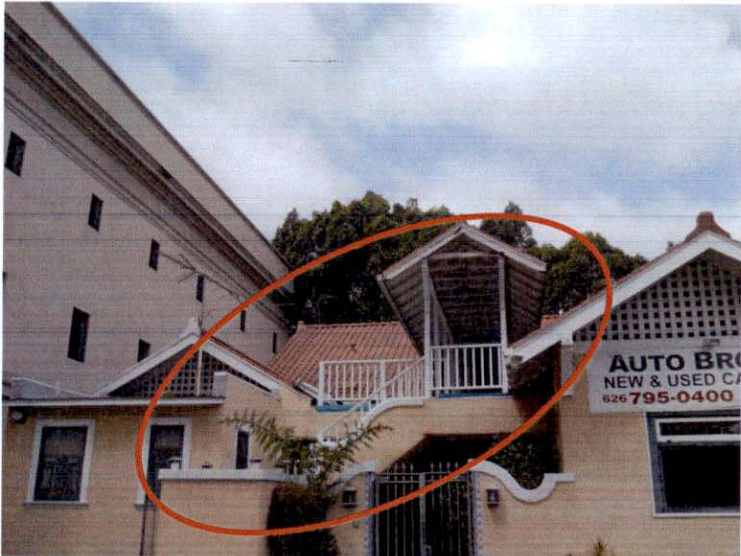
Figure 16: Non-Original Rear Stair and Walkway (Looking West)
