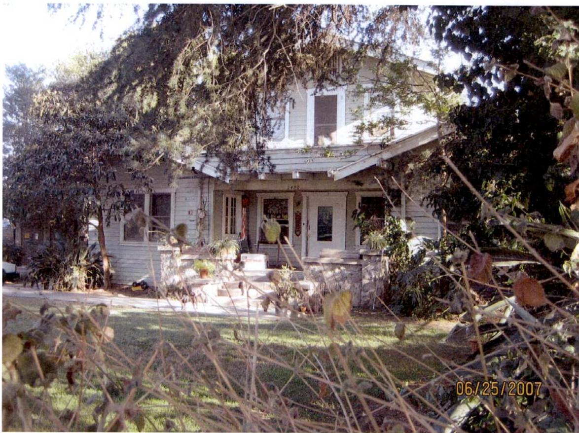
Attachment C: 2480 Oswego Street - 2007 Photo, North Elevation
