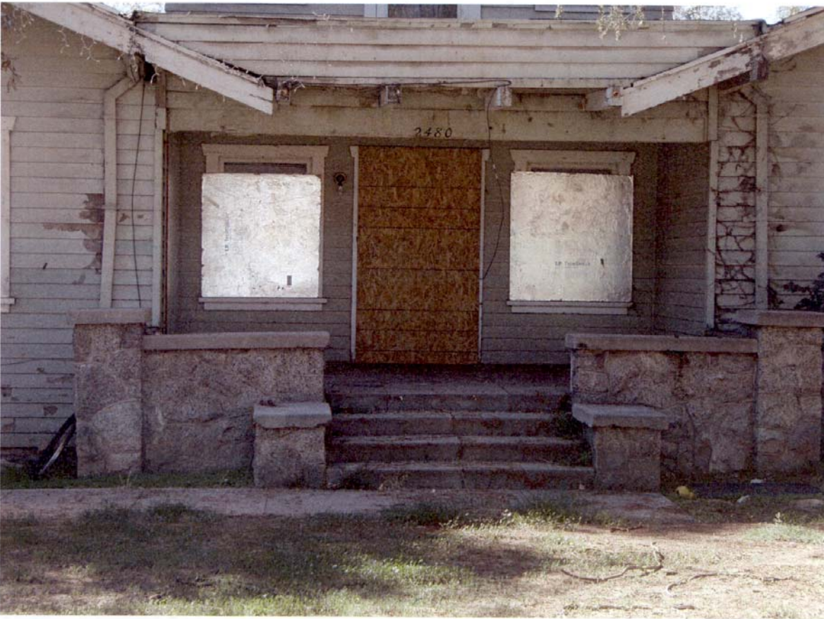
Attachment C: 2480 Oswego Street - Front Porch Detail
