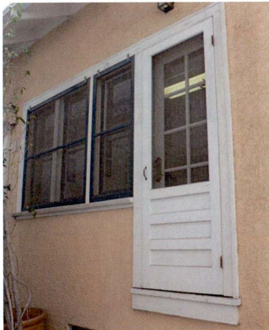
Figure 8. Looking northwest, south elevation, at a window opening resized for door opening; 1994 permit.
