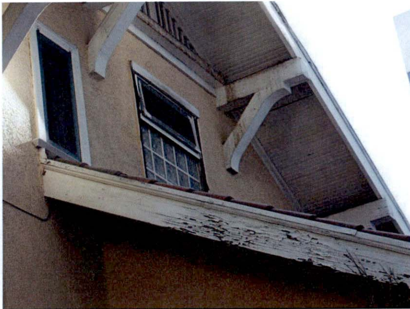
Figure 7. Looking northeast within the upper gable end showing an aluminum hopper window with glass-block window units.
