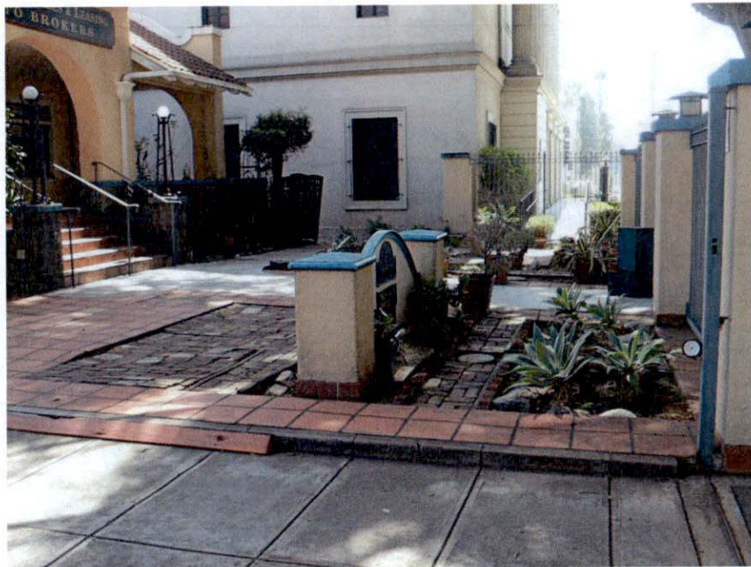
Figure 12. Looking south at the front yard area with modern Mexican tile porch pavers, concrete paving, red brick, and square piers with sign.
