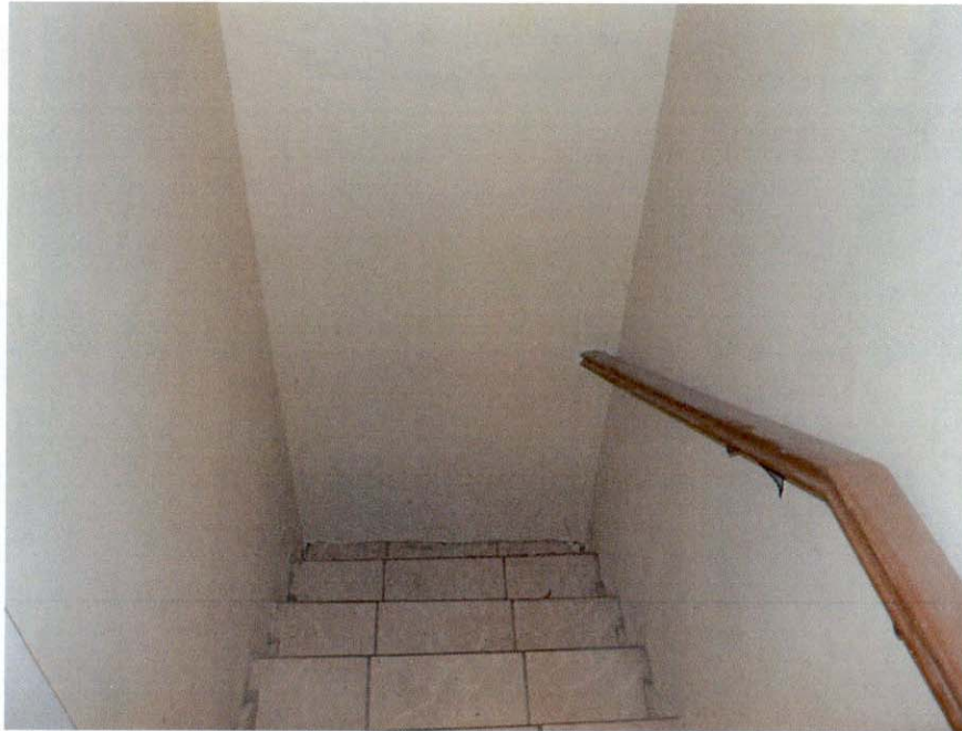
Figure 15. Looking south down the second-story stairs ending in a sealed wall closed off to the first floor.
