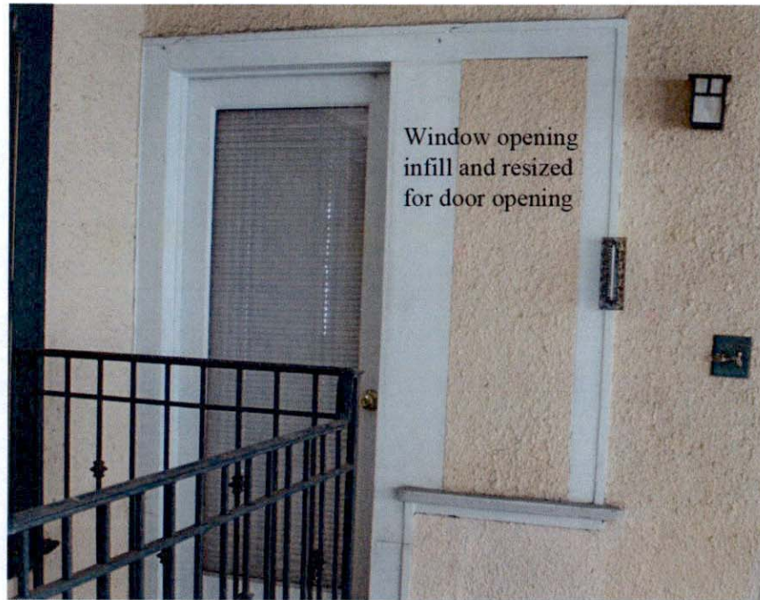
Figure 9. Looking north, south elevation of rear upper story, window opening infill and resized for door opening; 1994 alteration permit.
