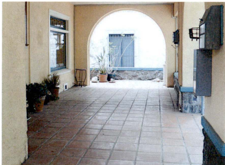
Figure 10. Looking south, main front porch replaced with Mexican tile porch pavers.
