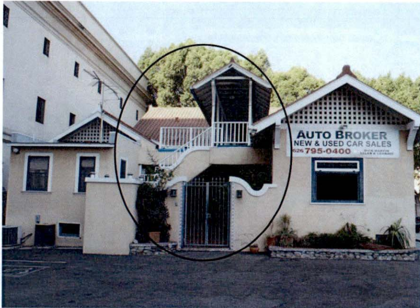
Figure 14. Looking west at the rear yard area showing the addition of stairs, upper porch and porch roof alteration.
