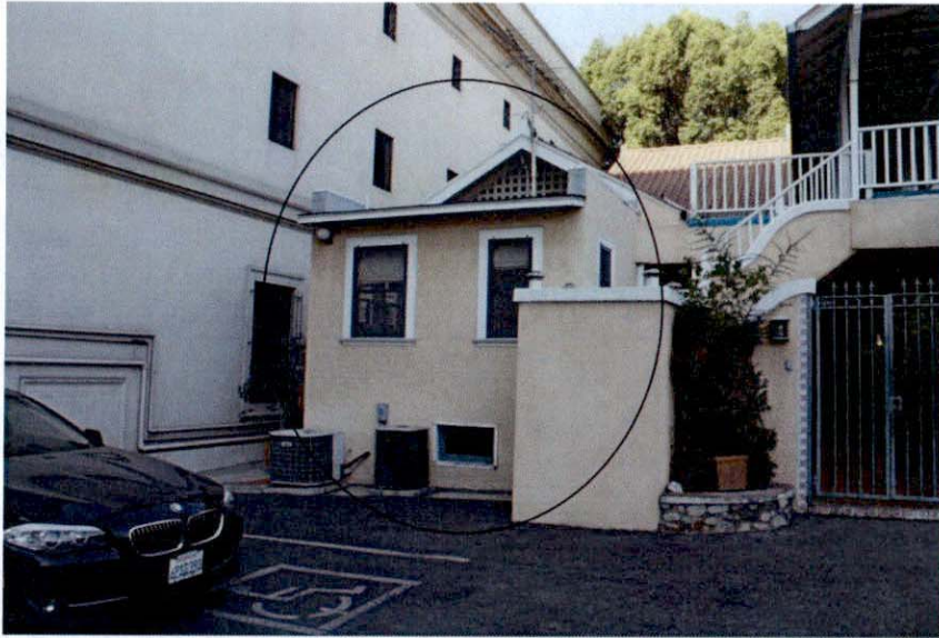
Figure 13. Looking southwest at the addition to the southeast corner of building.
