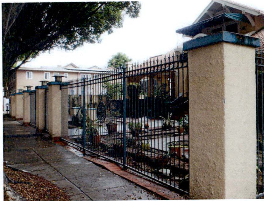
Figure 11. Looking northeast along the front yard area and sidewalk with six large piers and iron security fence.
