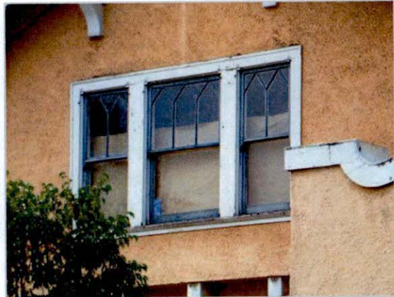
Figure 7: Original Windows on North Elevation. Source: GPA, November 2013.
