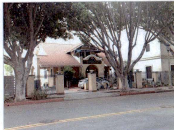
Figure 9: Context View Including Perimeter Fence. Source: GPA, November 2013.
