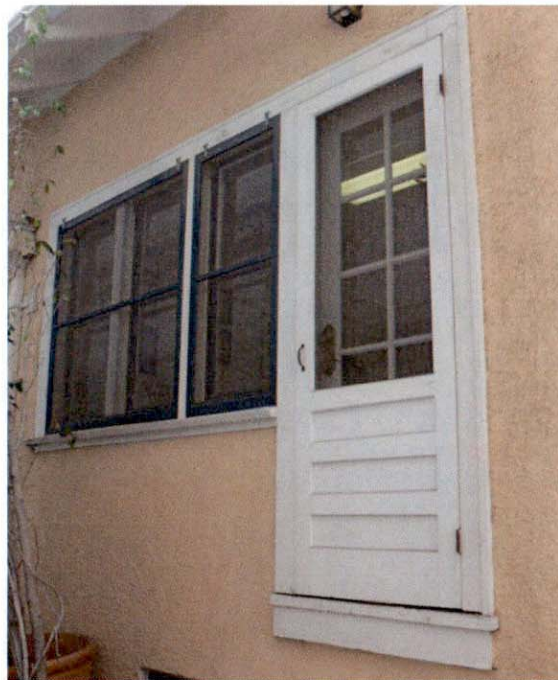
Figure 8. Looking northwest, south elevation, at a window opening resized for door opening; 1994 permit.
