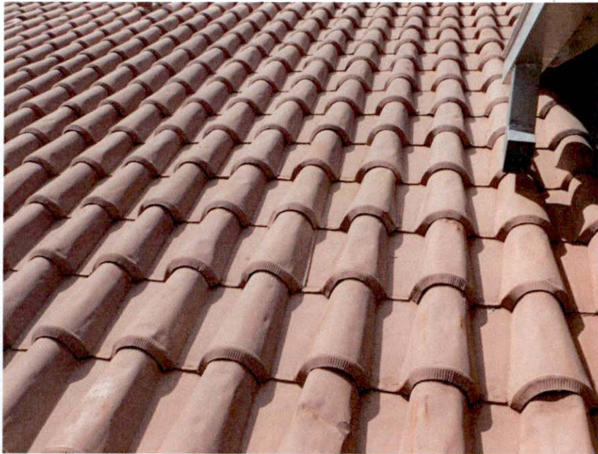
Figure 1. Looking east at the sheet metal roofing imitating a red clay tile roof, primary west elevation.
