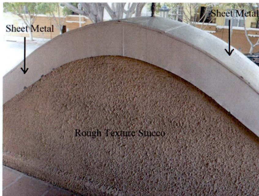
Figure 2. Looking west, within upper porch, at the sheet metal coping over parapet with a rough texture stucco wall surface.
