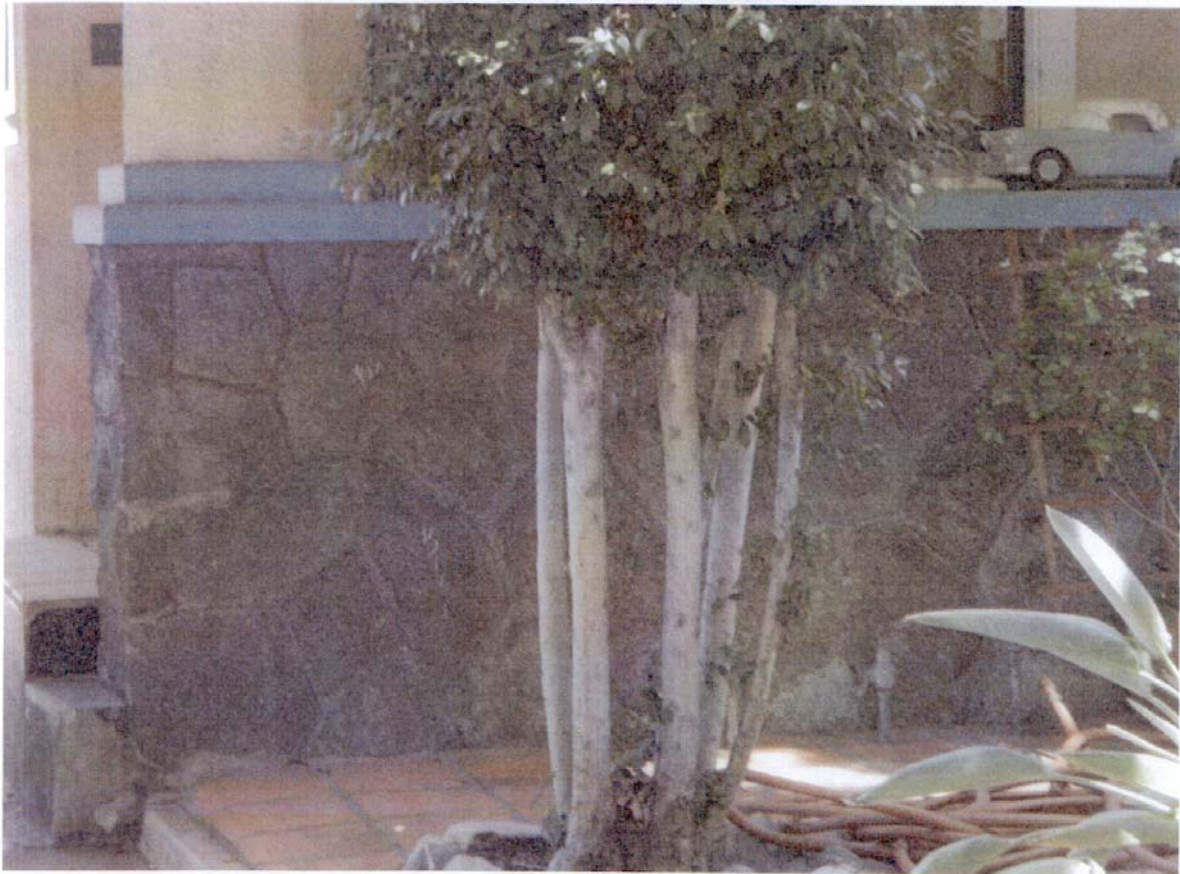
180 S. Euclid Avenue Rock Porch Wall Detail
