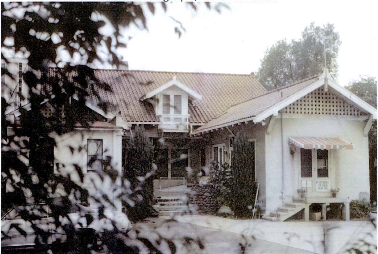
180 S. Euclid Avenue 1979 Photograph; East Elevation
