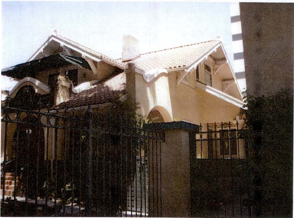
180 S. Euclid Avenue West and South Elevations
