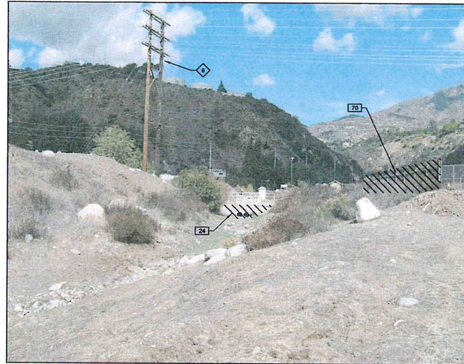
1 DEMOLITION PHOTO 1 SCALE: NO SCALE FILE: FILE
