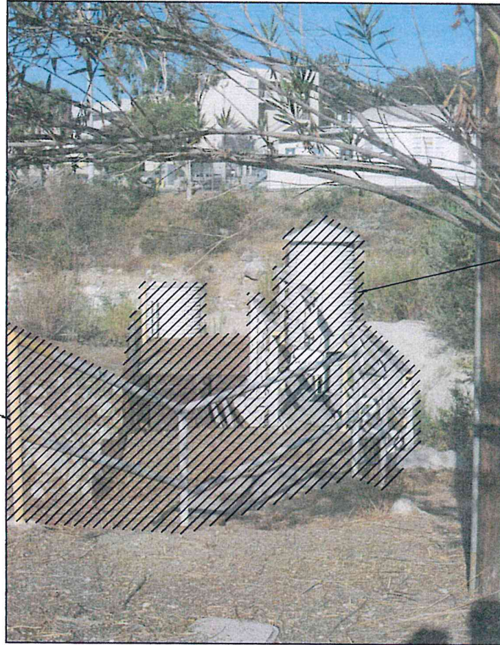
6 DEMOLITION PHOTO 6 03D-02 SCALE: NO SCALE FILE: FILE
