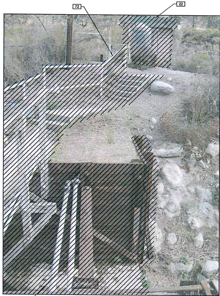
3 DEMOLITION PHOTO 3 03D-02 SCALE: NO SCALE FILE: FILE
