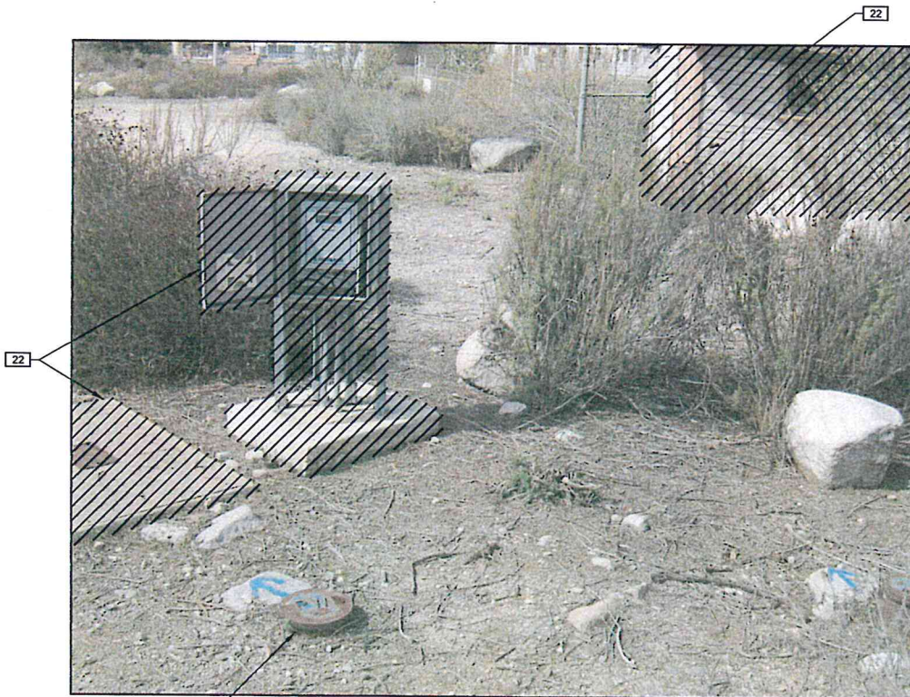
5 DEMOLITION PHOTO 5 03D-02 SCALE: NO SCALE FILE: FILE
