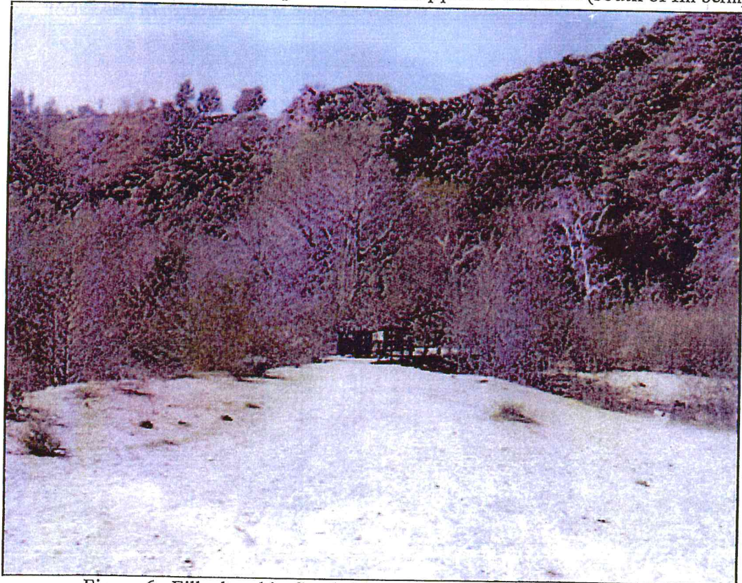
Figure 6. Fill placed in floodplain to access headworks structure.
