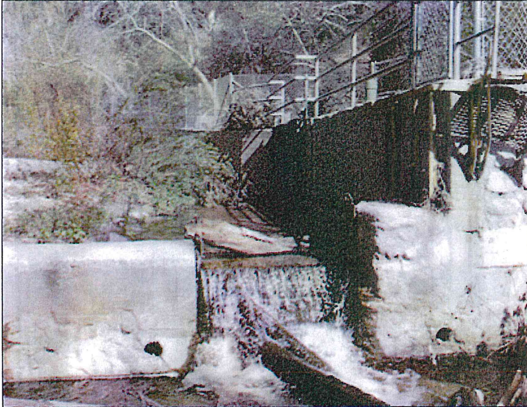
Figure 7. Existing diversion dam in Area 2.
