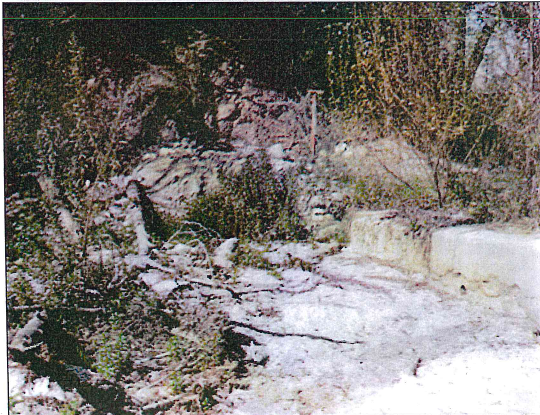
Figure 8. Wildlife can easily pass over and around existing diversion structure in Area 2.
