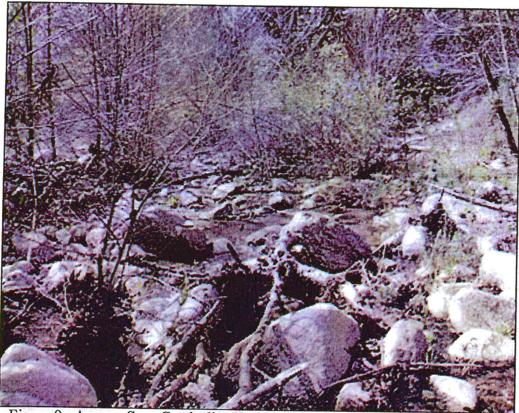
Figure 9. Arroyo Seco Creek directly below the existing diversion structure.
