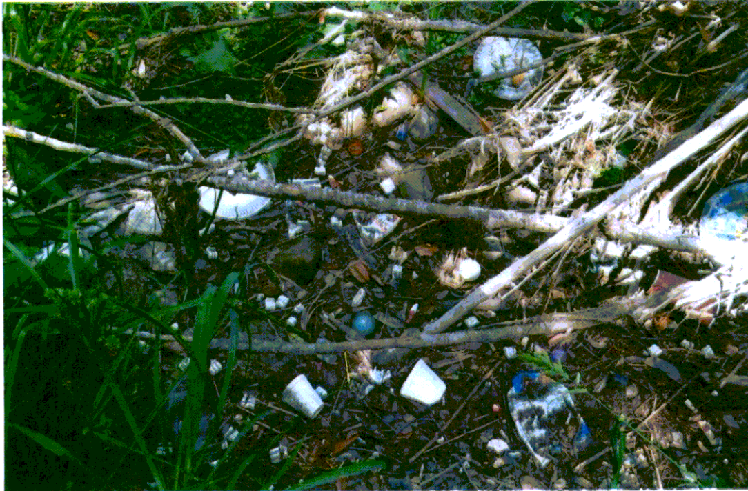
Polystyrene trash caught under Colorado St. Bridge (courtesy of Tim Martinez)
