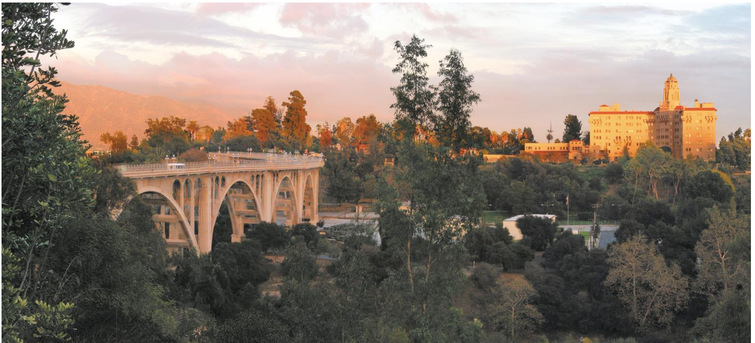
View of the Colorado Street Bridge
