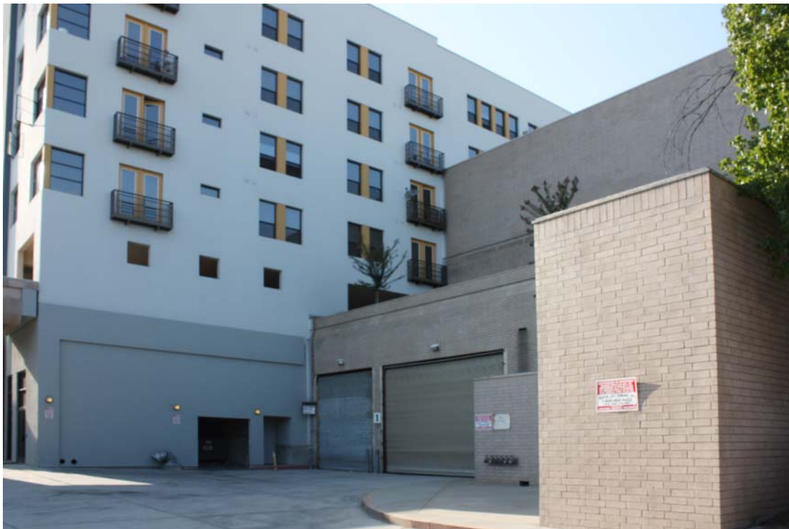
Figure 11: View northwest of juncture of Macy's store and Paseo Colorado apartments (south façade on E. Green Street). (ARG, 9/19/2013)
