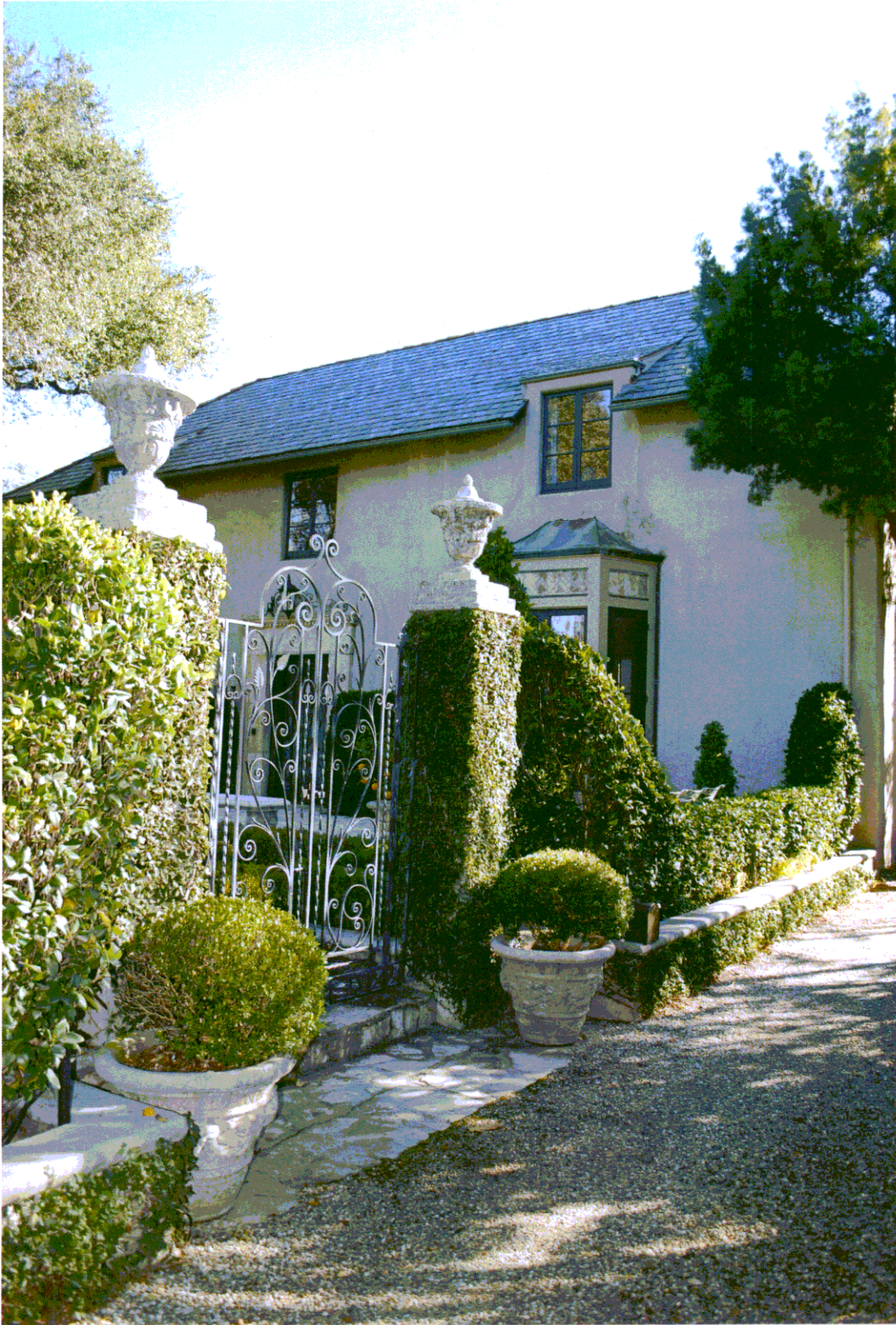
Non-Historic Pilasters & Gates along Driveway
