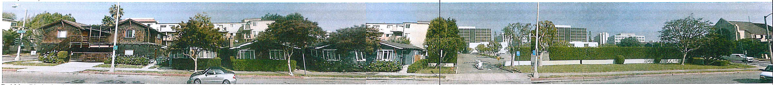
Del Mar Blvd. viewing North, towards site
