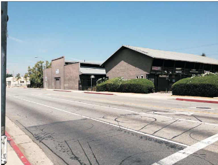
Photograph 3: Northwesterly view of on-site vacant Davis Lumber buildings.
