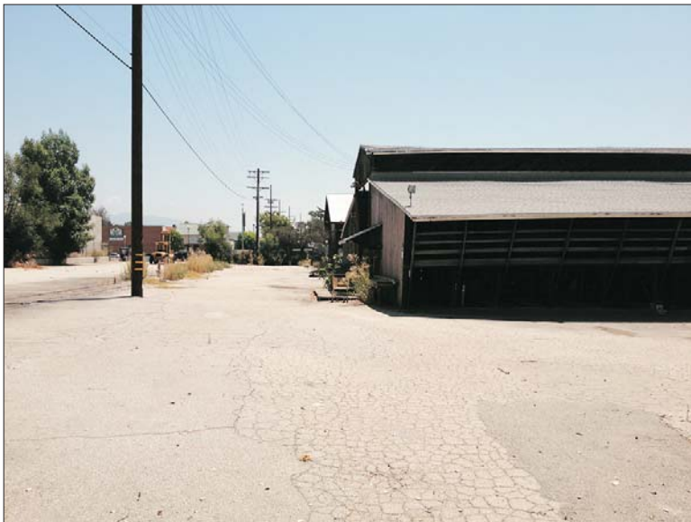
Photograph 7: Easterly view of on-site vacant Davis Lumber buildings.
