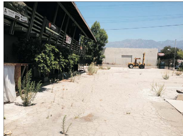
Photograph 8: Northerly view of on-site vacant Davis Lumber buildings.
