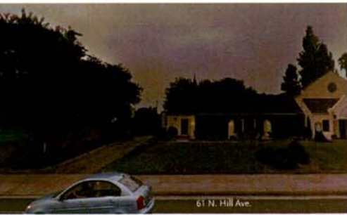
View of the church to the North of the Proposed Project along Hill Ave. 7
