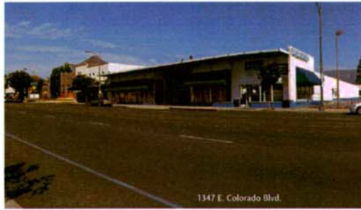
View of existing buildings on North Parcel site from Colorado Blvd. 4
