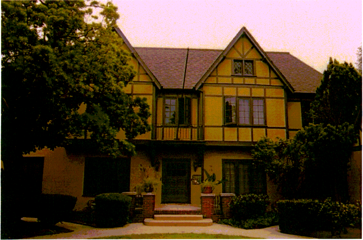
Rear fourplex building - front view
