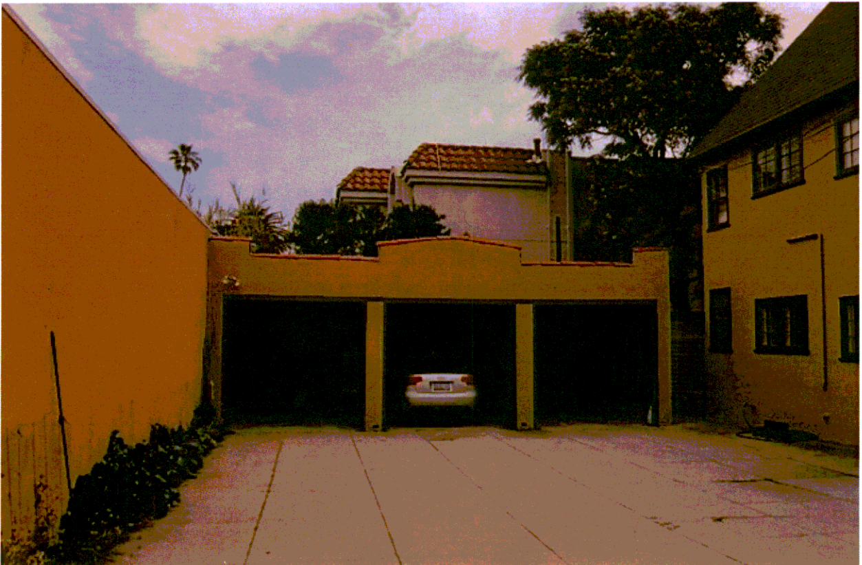
View of rear carport
