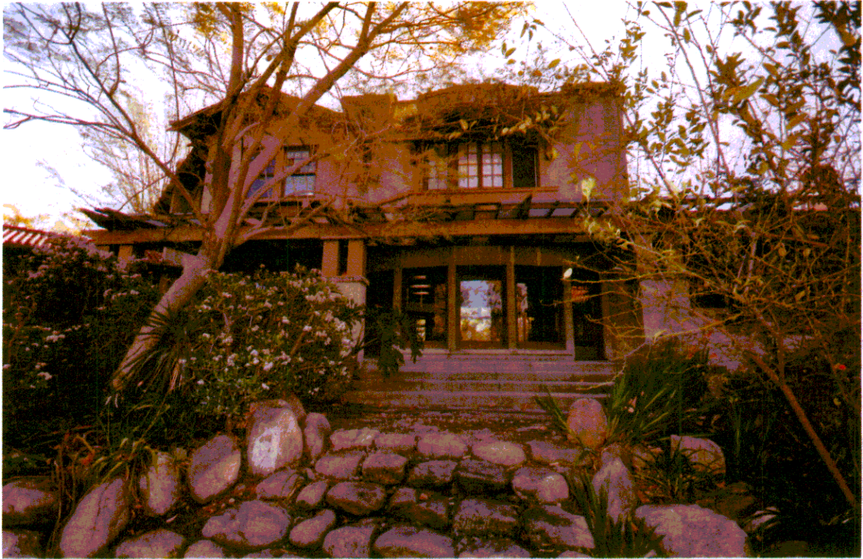
7 - Northwest elevation, Lkg SE
