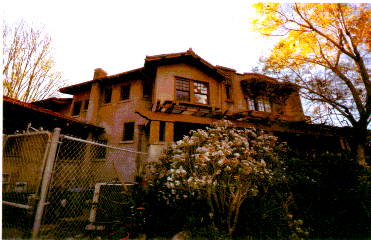
6 - North elevation, Lkg SE
