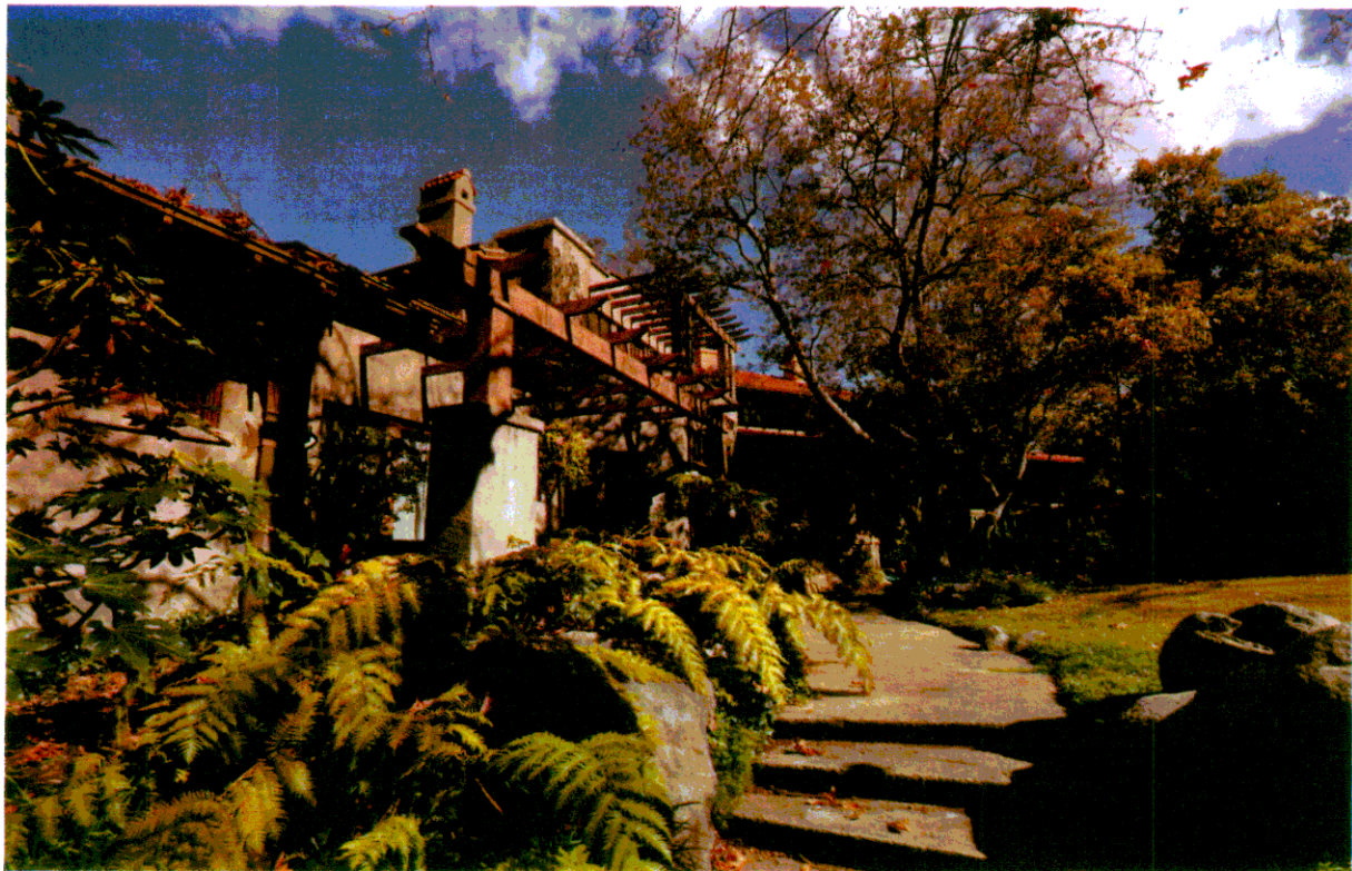
10 - Southeast elevation, Lkg NE
