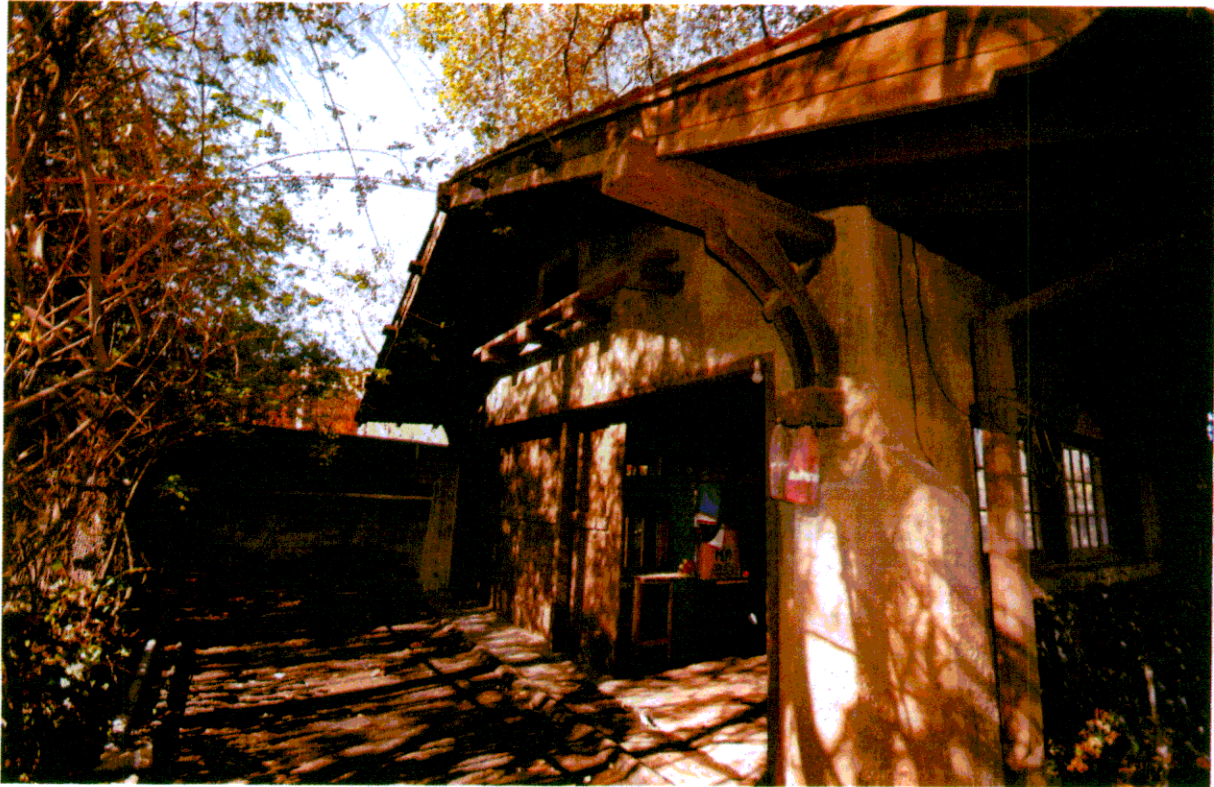
47 - Detached garage, Lkg NW
