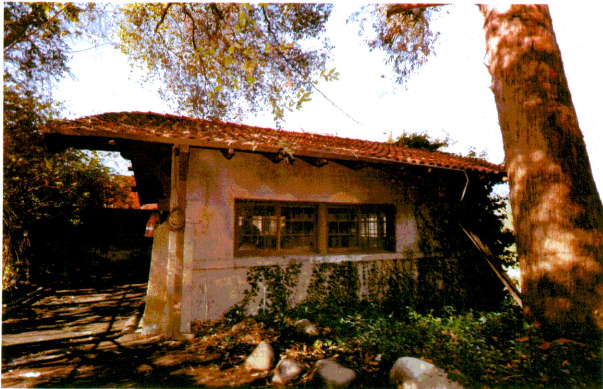
48 - Detached garage, NE elevation, Lkg SW
