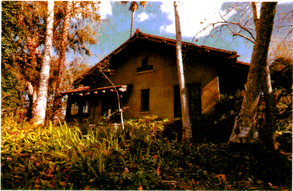
9 - Southwest elevation, Lkg NE
