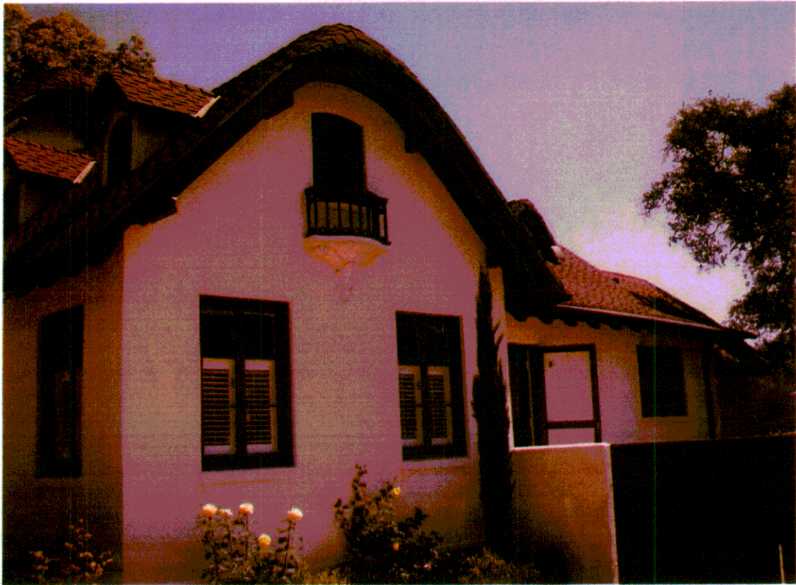
South elevation facing Northeast
