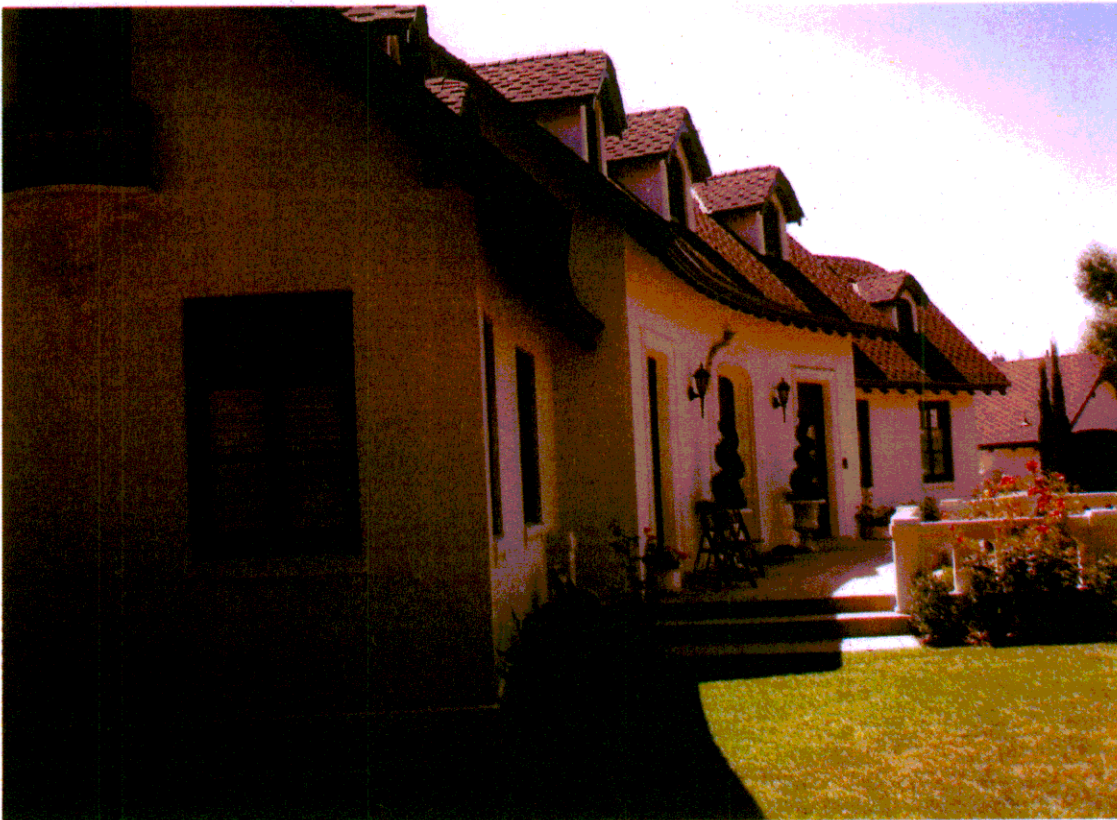
West & North elevations facing south
