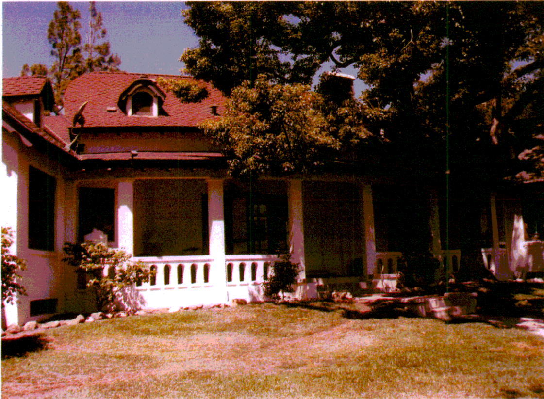
East (rear) elevation facing west
