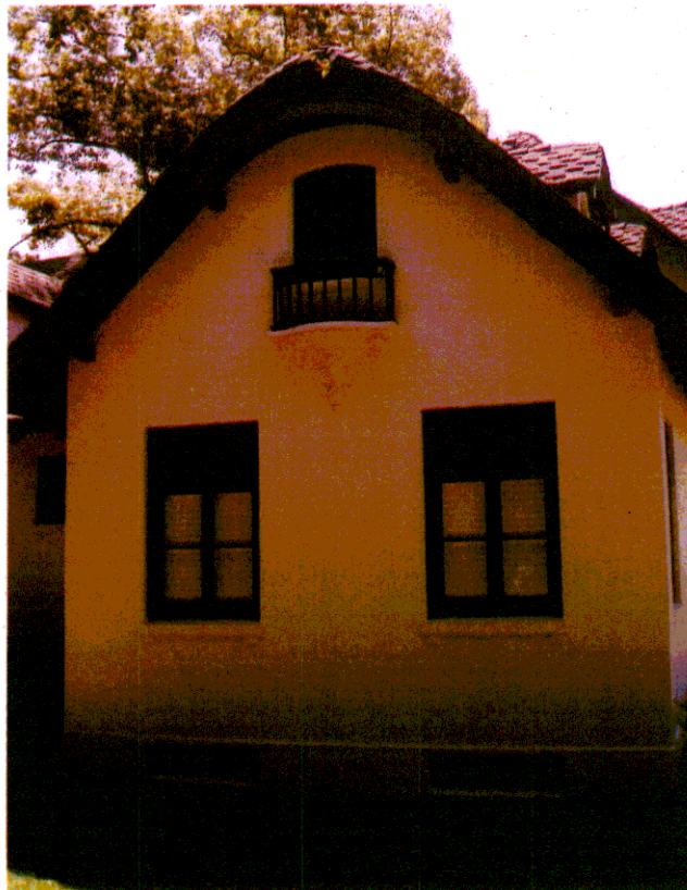
North elevation facing south
