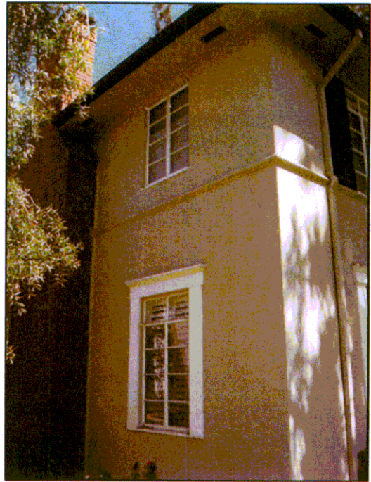
Window detail and chimney
