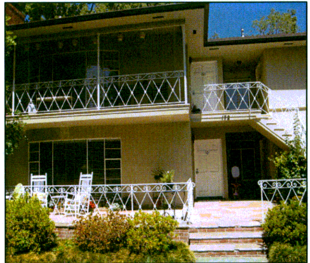
Courtyard elevation, balcony, ironwork
