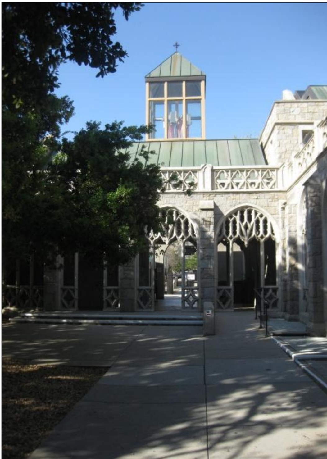
View from within All Saints Church complex courtyard looking north towards project site. 1970s era breezeway and cupola behind arcade are slated for removal.
