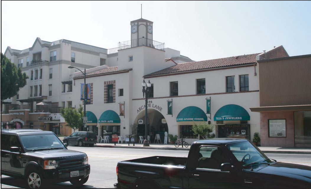
Photo 1 - View of adjacent development to the east on Colorado Boulevard. The existing project site structure is partially visible in the right side of the frame. The Arcade Lane building is directly adjacent.
