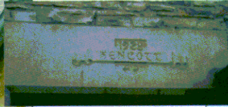
Lintel at Front Door
