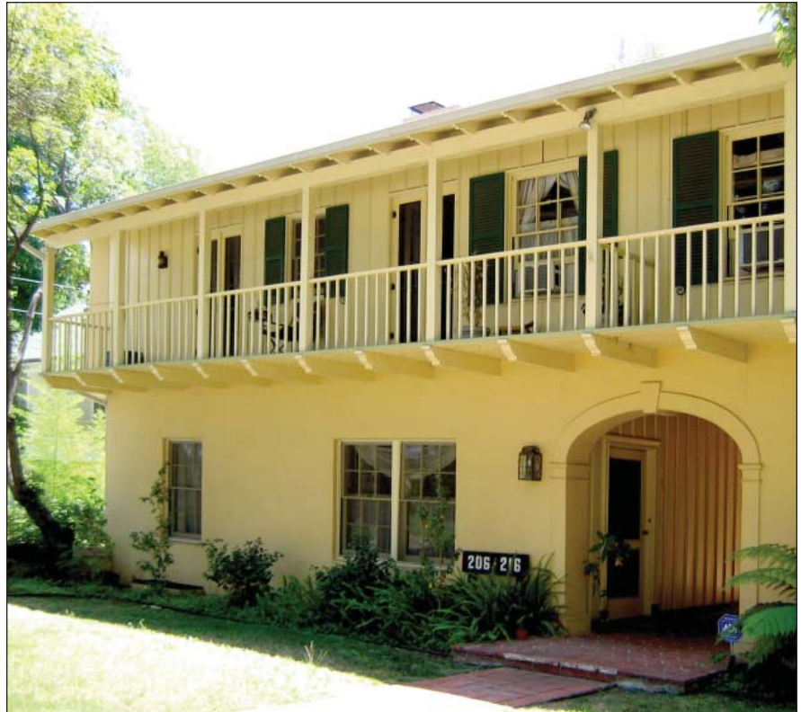
(Right) Units to this courtyard building are accessed through an inviting, prominently located covered passage (zaguan).
