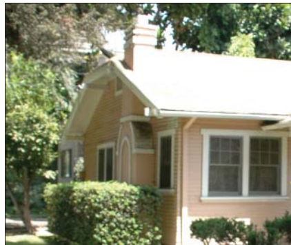
H. Attached chimney
