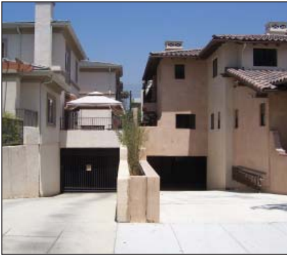
(Above) ⚠️ The adjacency of these two multi-family residential parking entrances creates an unfortunate expanse of driveway and two large garage openings. The misaligned planter wall that separates them as well as the mismatch in the size of the two respective openings compounds the problem.
