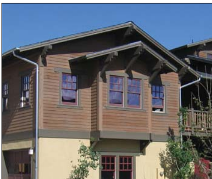
A. Cantilevered bay window
