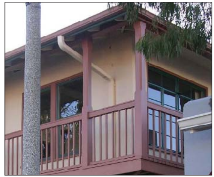
F. Gutter and downspout internal to balcony
