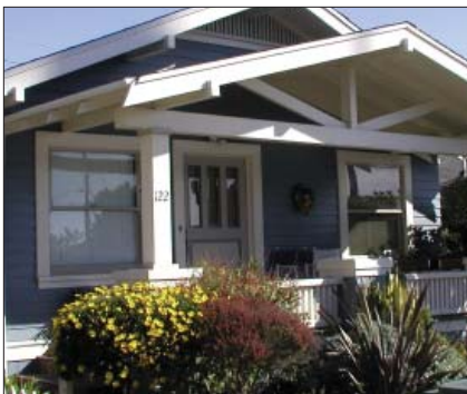
G. Single opening and door with lights.
