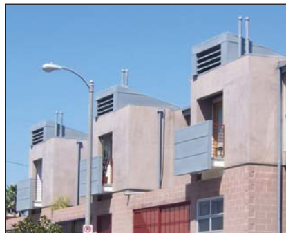
Roof vents integrated into a multi-family building's facade design. The vents are grouped together and repeated in a serial rhythm.
