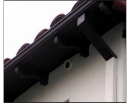
F. Gutter painted to match eave and walls.
