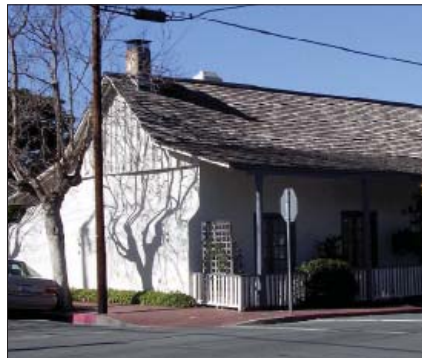
E. Shingle roof with compound slope.
