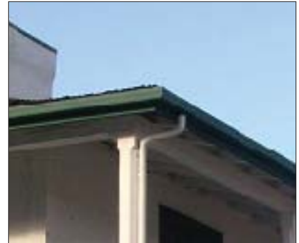
F. Gutter and downspout external to balcony
