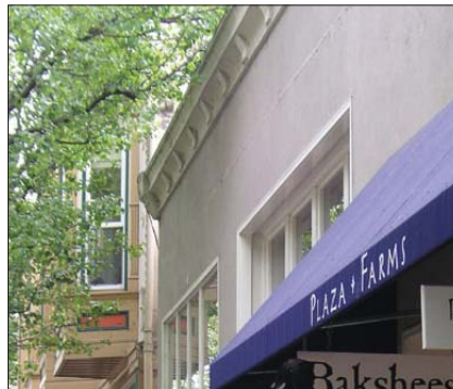
E. Parapet with decorated cornice
