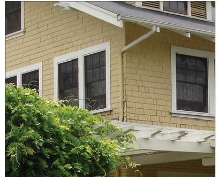
F. Gutter and downspout
