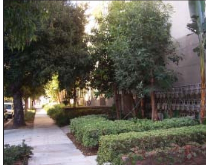
⚠ A bank of gas meters that is completely visible from the street and sidewalk.
