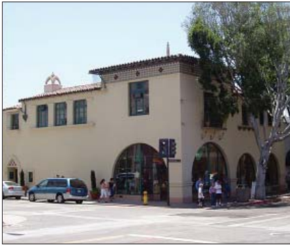
A. Tower at corner
