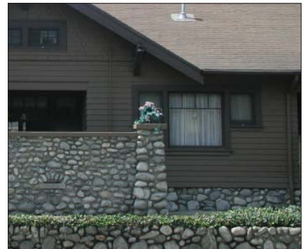
C. Stone base with clapboard siding
