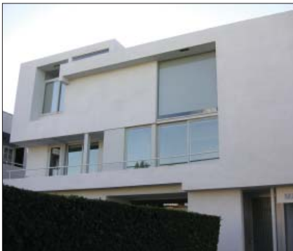
D. Irregular roof profile
