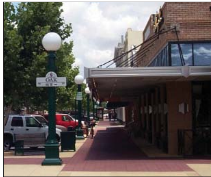
H. Canopy supported by cables.
