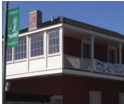
H. Cantilevered balcony, partial enclosure
