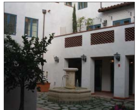
C. Plaster walls with clay tile grills
