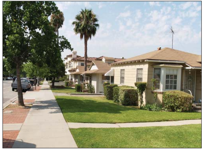
A residential street with a public realm character comprised of consistent setbacks and compatible massing.
