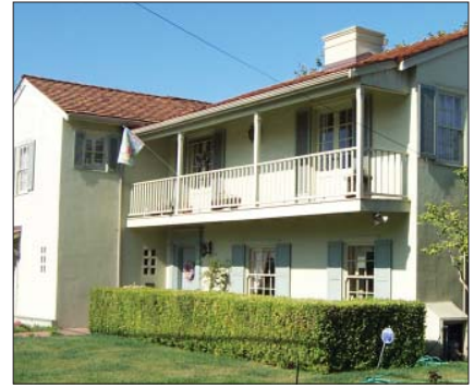
C. Plaster walls extend to two stories
