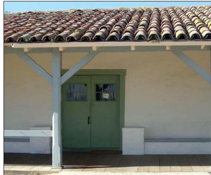
E. Sloped tile roof over building and porch
