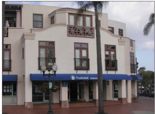
A mixed-use building clad in plaster. The moldings and column bases are constructed of durable materials (precast concrete and tile, respectively).
