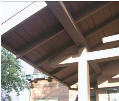
D. Exposed rafter tails
