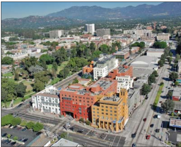
The relationship among adjacent buildings defines the character of a block.
