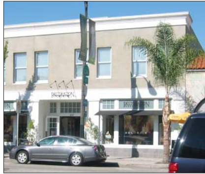
E. Flat roof with simple, street-facing cornice
