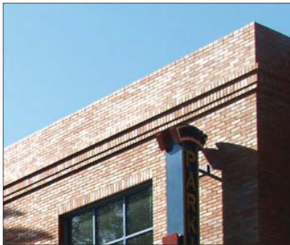
D. Brick cornice line
