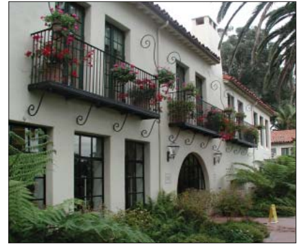
C. Plaster walls with formal window composition
