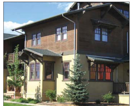
C. Plaster and wood siding
