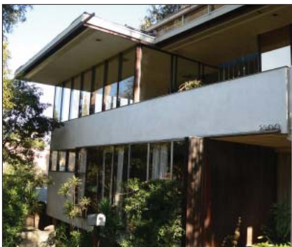
D. Cantilevered roof protecting windows
