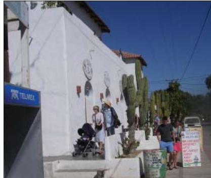
E Parapet with flat roof
