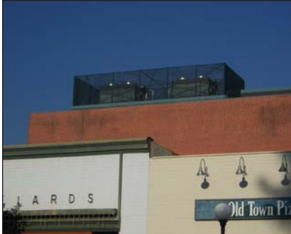
⚠ Screening that does not hide the mechanical equipment.
