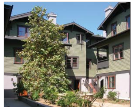
I. Courtyard planted with large tree.
