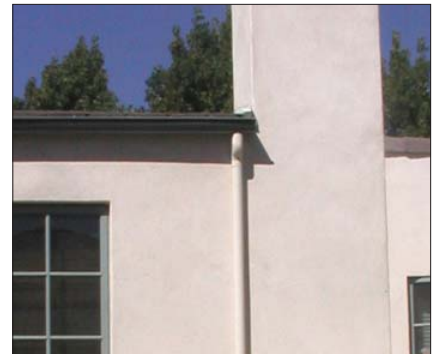
F. Gutter and downspout
