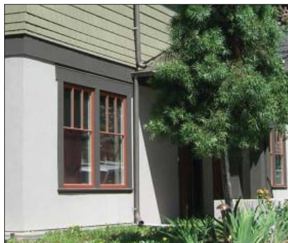
B. Plaster ground floor as base.
