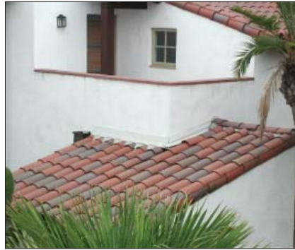
E. Sloped tile roof
