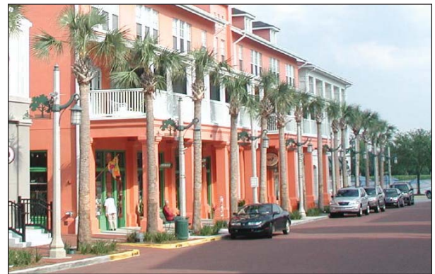
A mixed-use commercial building with a gallery frontage.
