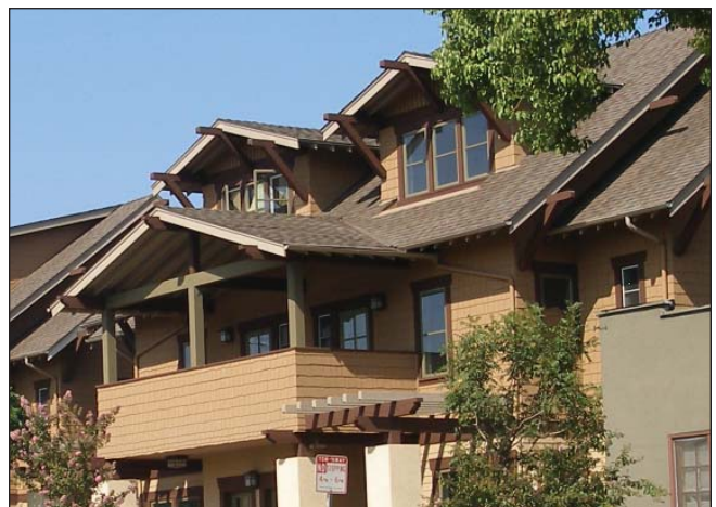
Upper floors are incorporated into attic spaces and are daylit by dormer windows.
