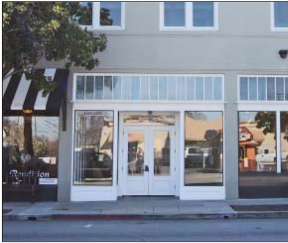
G. Shopfront openings with transom windows
