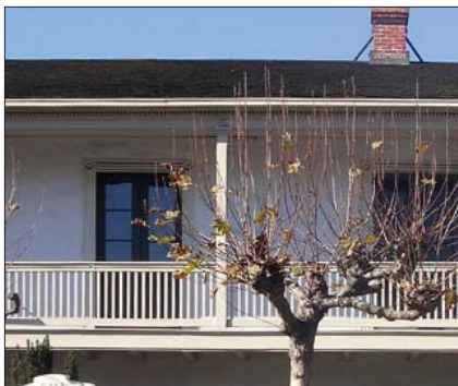
D. Articulated wood beam and shingles
