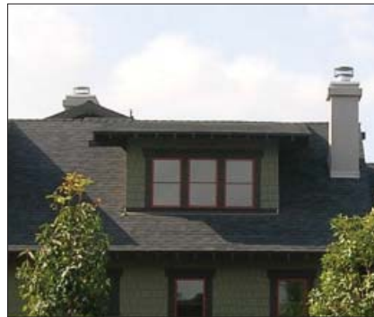
E. Dormer with shed roof.
