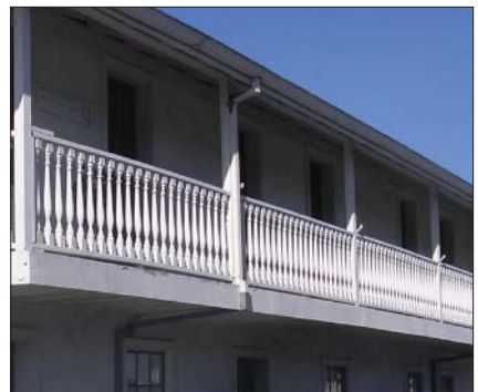
F. Gutter and downspout external to balcony
