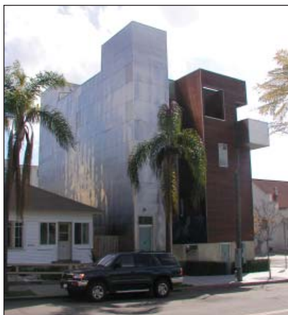
(Above) ⚠️ This multi-family building, through its size, massing, lack of windows, and use of reflective cladding, overwhelms its existing neighbor.
