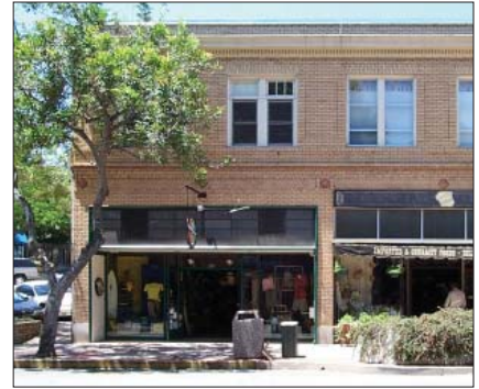
C. Multi-colored brick walls
