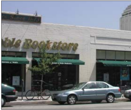
D. Brick wall extended as parapet
