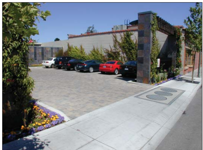
A commercial parking lot that includes planting areas and semi-permeable paving to facilitate rainwater recharging.
