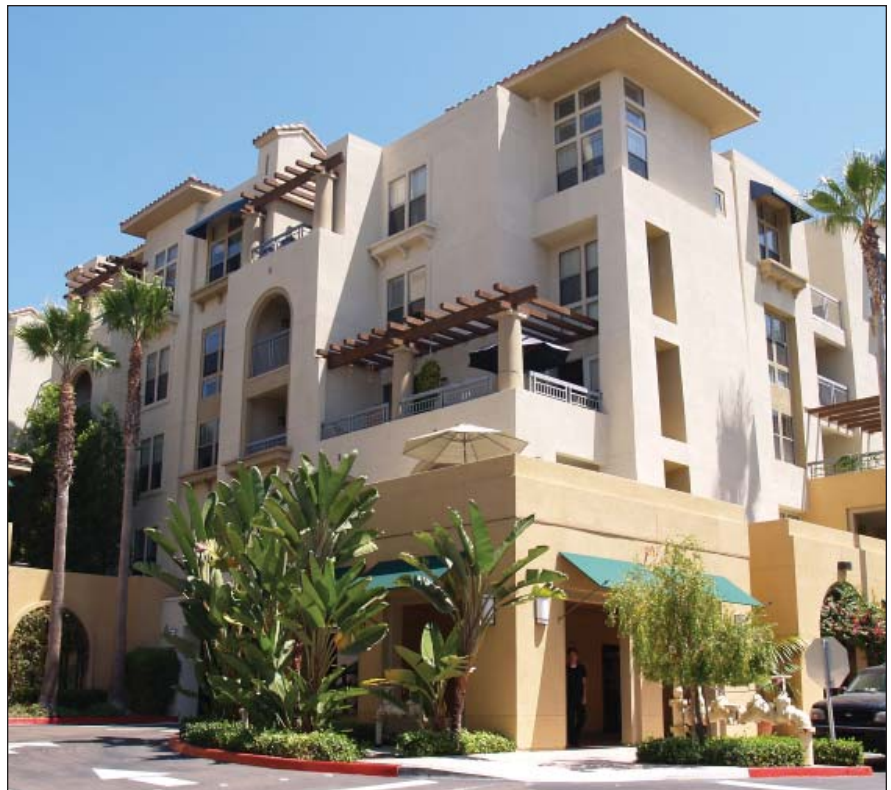
(Right) A multi-family building that responds to Southern California's climate through the use of large overhangs, trellises, and canopies to shade window openings and to provide inviting outdoor spaces.
