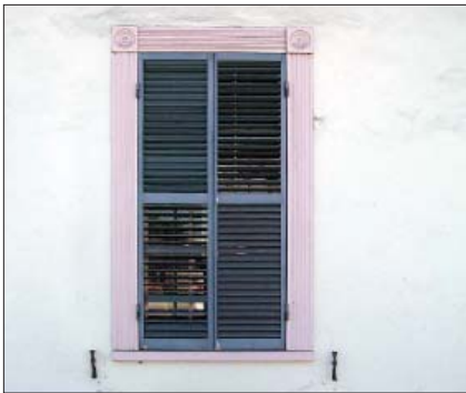
G. Elaborate trim with closed, louvered shutters
