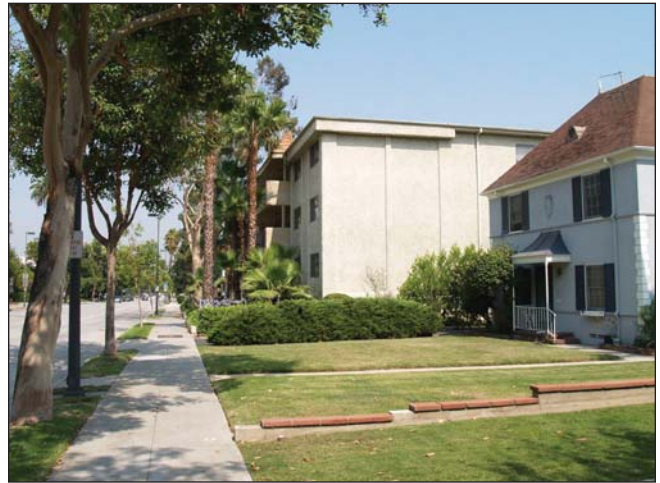
⚠️ A residential street with a public realm character comprised of inconsistent setbacks and incompatible massing.
