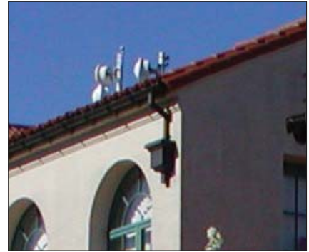
F. Gutter transitions to internal drain pipe.
