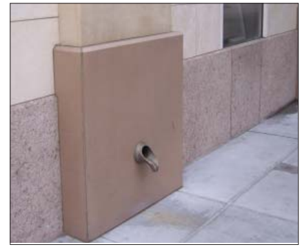
F. Internal roof drains
