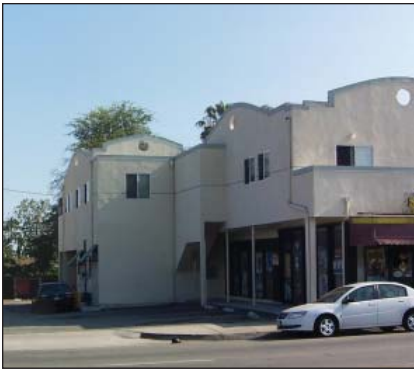
(Above) ⚠️ While the ground-floor retail uses are accessed directly from the sidewalk, there is no indication here as to how the second-floor residential units are accessed.
