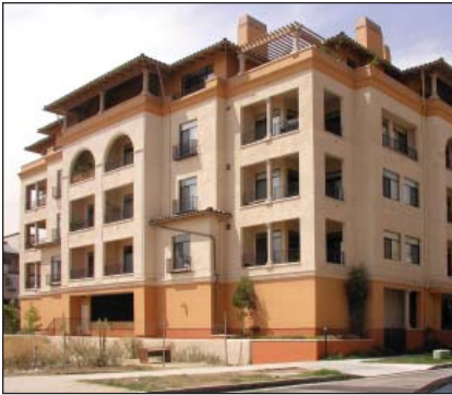
⚠ An above-ground parking garage with blank walls facing a neighboring property.
