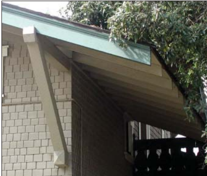
D. Wood brace and exposed rafters.
