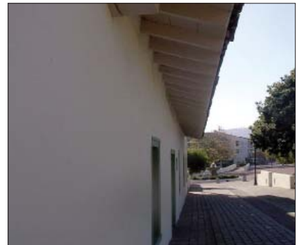
C. Rustic plaster
