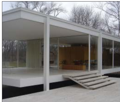
B. Building disengaged from ground.
