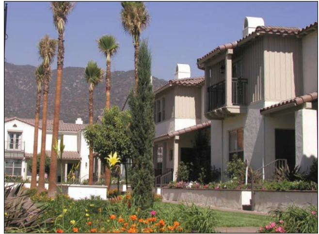
A multi-family building clad in plaster and fiber-cement siding. The vertical transition between the plaster and siding occurs at the inside corners.
