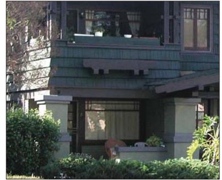
C. Painted shakes above painted plaster
