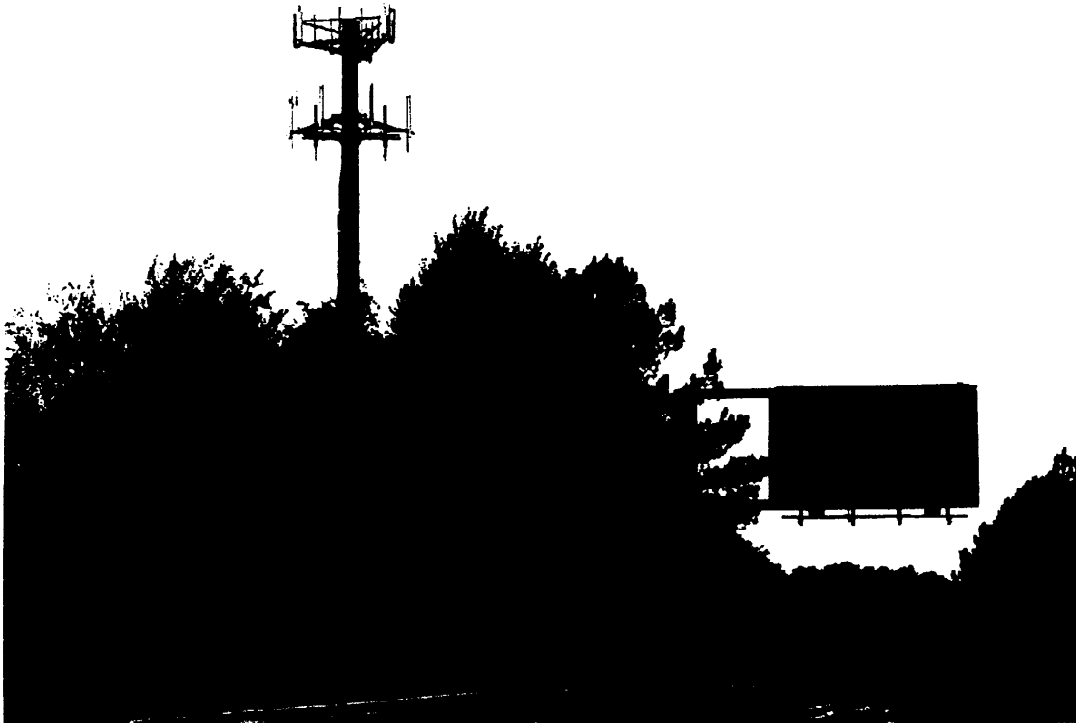
Figure 3: Uncamouflaged Monopole wireless site in Fairfax, Virginia.
