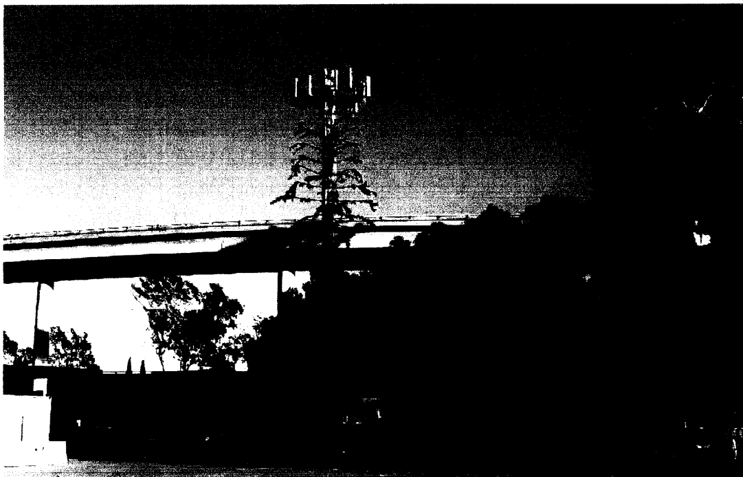
Figure 6: Inferior Monopine wireless site in Los Angeles, California.
