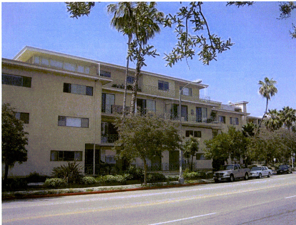
“Whispering Waters” 1000 Cordova Street, Pasadena, CA 91106 East Building north (front) façade with East Penthouse, looking southwest May 23, 2005
