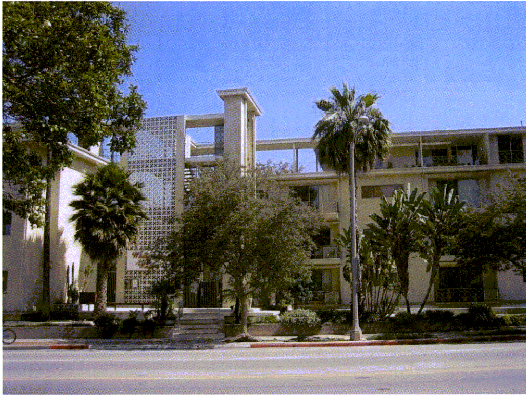
“Whispering Waters” 1000 Cordova Street, Pasadena, CA 91106 Center of north (front) facade, looking south May 23, 2005
