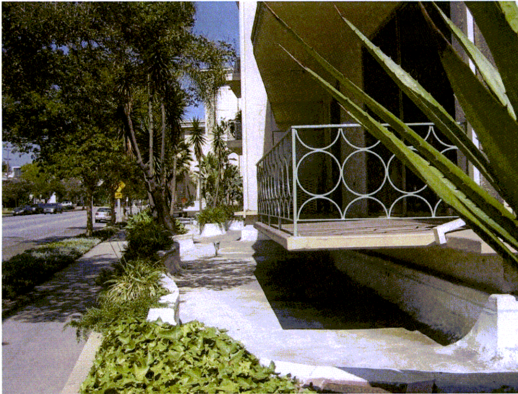
“Whispering Waters” 1000 Cordova Street, Pasadena, CA 91106 Waterfeature West Building end of building, looking east May 23, 2005
