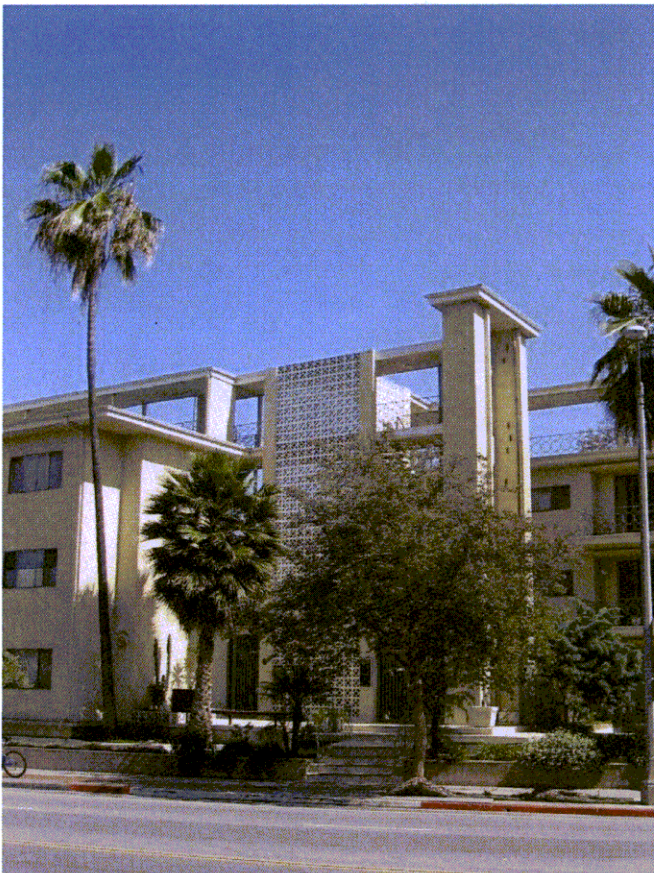
“Whispering Waters” 1000 Cordova Street, Pasadena, CA 91106 Central Tower (detail) north (front) façade easterly view looking southeast May 23, 2005
