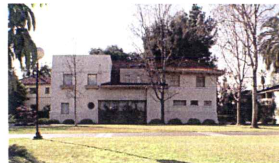
4B - Library Annex
