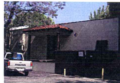
3B - Landscape - bldg 25 (demolished)
