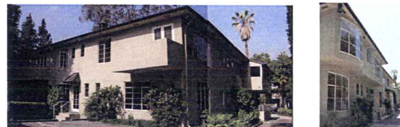
3 - South Orange Grove Apartments-bldg 35 & 39
