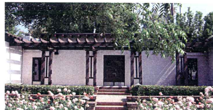
4B - Health Center - bldg 21 (demolished)
