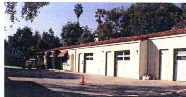
3C - Villa Francesca Garage - bldg 26 (demolished)
