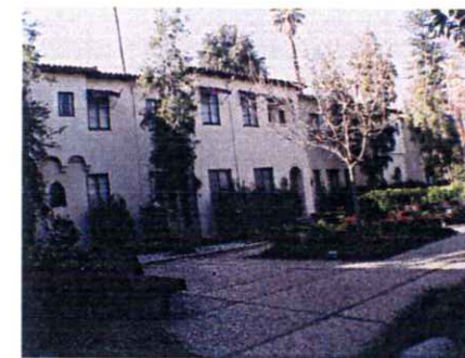
3A - Grove Manor - bldg 24
