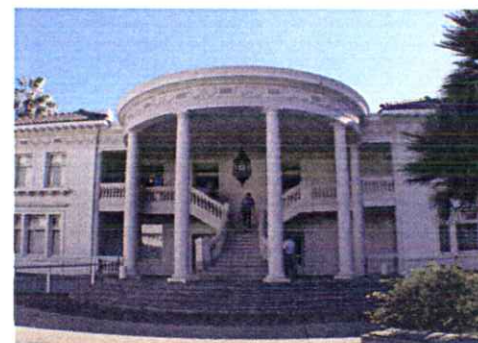
2A - Merritt Mansion-bldg 41
