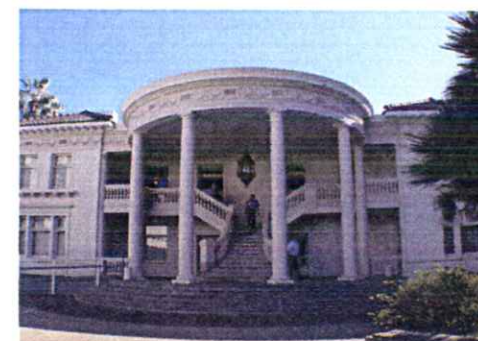
2A - Merritt Mansion-bldg 41
