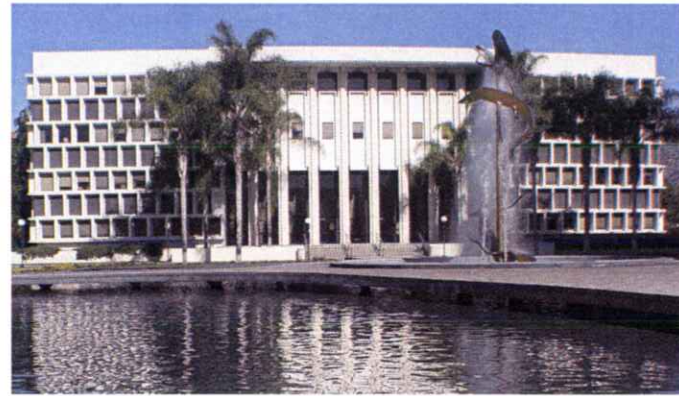
2 - Hall of Administration -bldg 62 (demolished)
