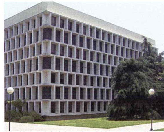
1b - Hall of Administration -bldg 62 (demolished)
