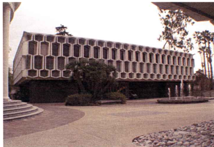
4c - Science Hall-bldg 43 (demolished)
