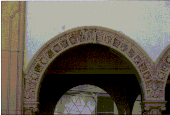
Entry arch/capital detailing
