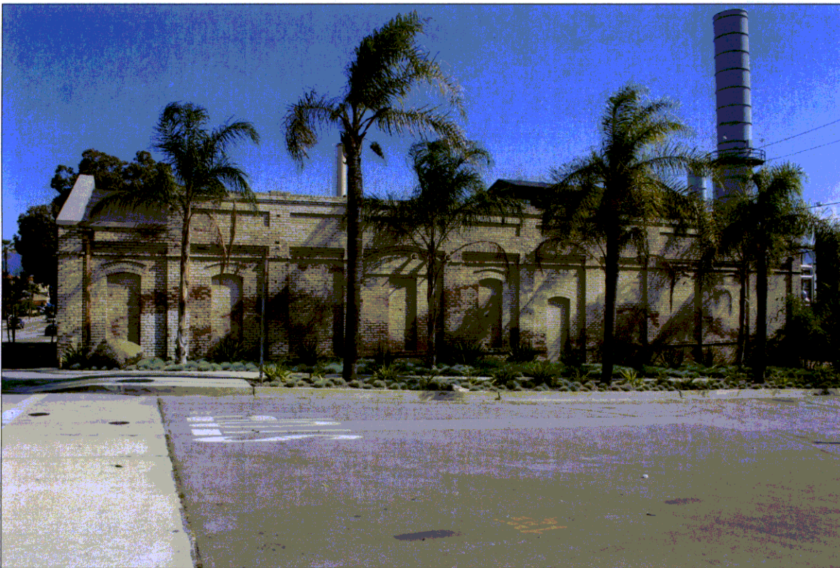
State Street elevation - current
