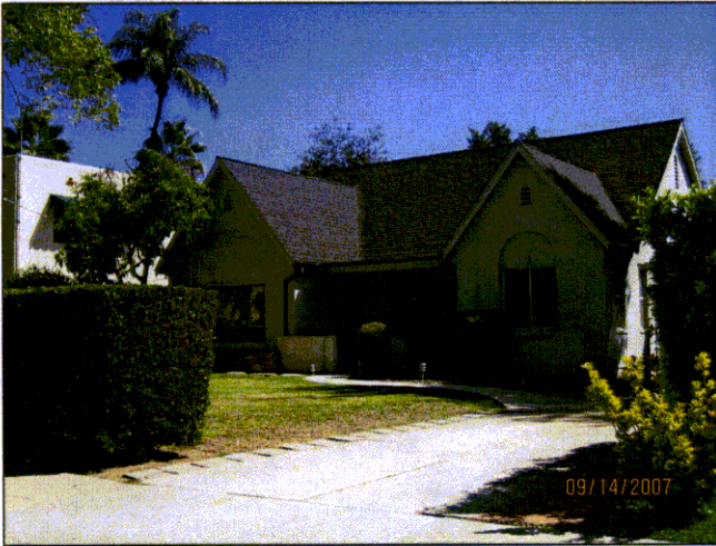
940 Atchison Street, 1925, F.R. Finch
