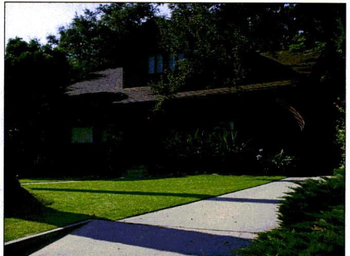
979 Atchison Street, 1908, Arch. Design Co.
