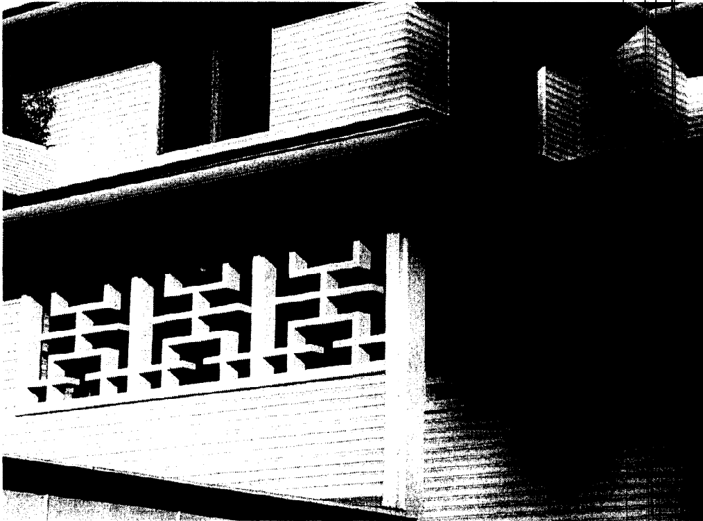
Figure 2--Front elevation, note the two different window screen types.
